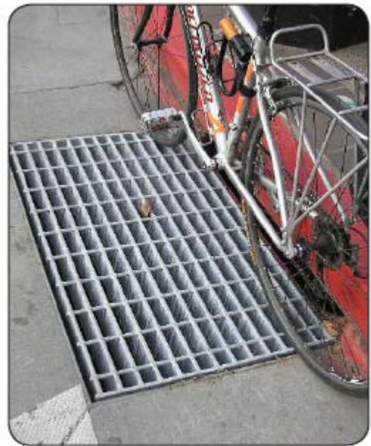
Examples of bicycle-safe drainage grates.
