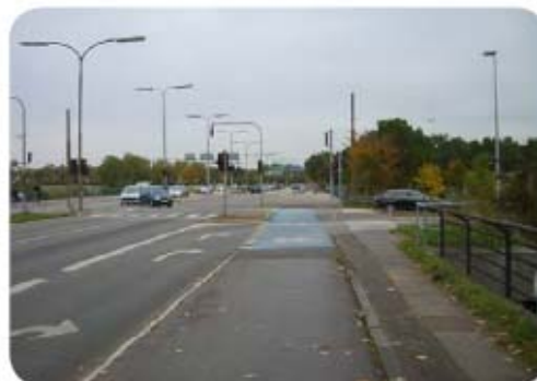
At this unsignalized right turn, the cycle track has dropped to a bike lane with blue coloration and pavement markings through the conflict area.
