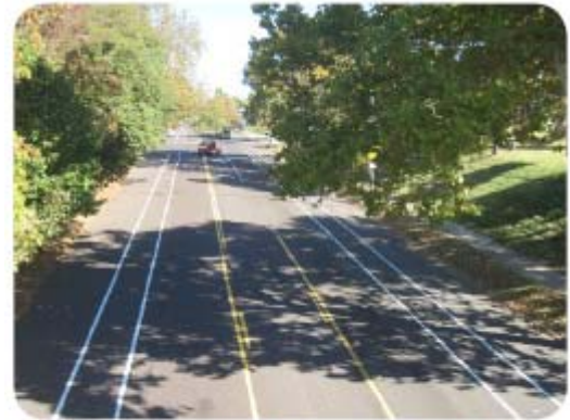
This road was re-striped to convert four vehicle travel lanes into three travel lanes with bike lanes.
