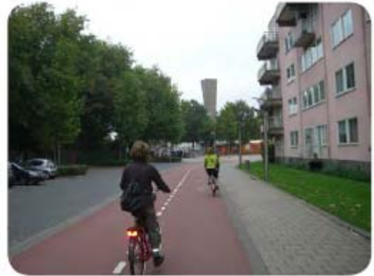
Two-way cycle track with dividing line.
