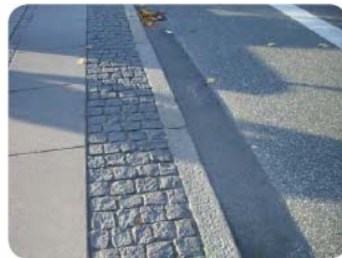
Mountable curb, Copenhagen.
