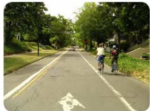
This contraflow bike lane in Portland, OR (left) provides a key connection along a narrow one-way street.
