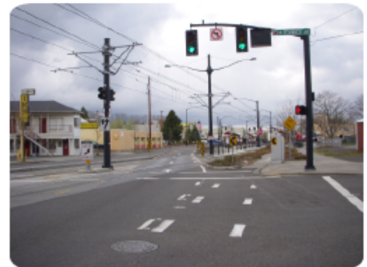
Bike lane dashed through complex intersection.
