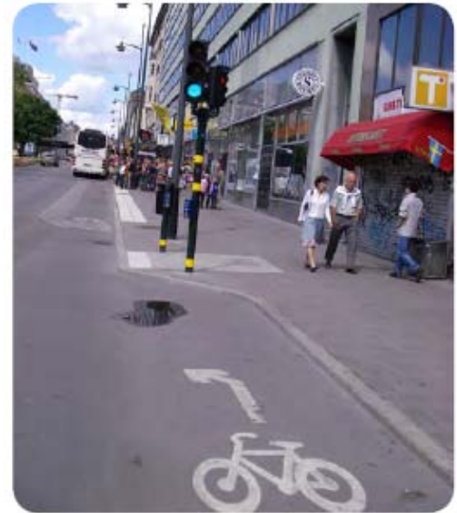
Left-turn from a cycle track on the right via bicycle-signal phase in Stockholm, Sweden.
