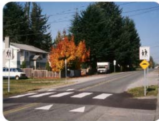
Speed humps are a common traffic calming treatment, which should not be used on emergency routes.
