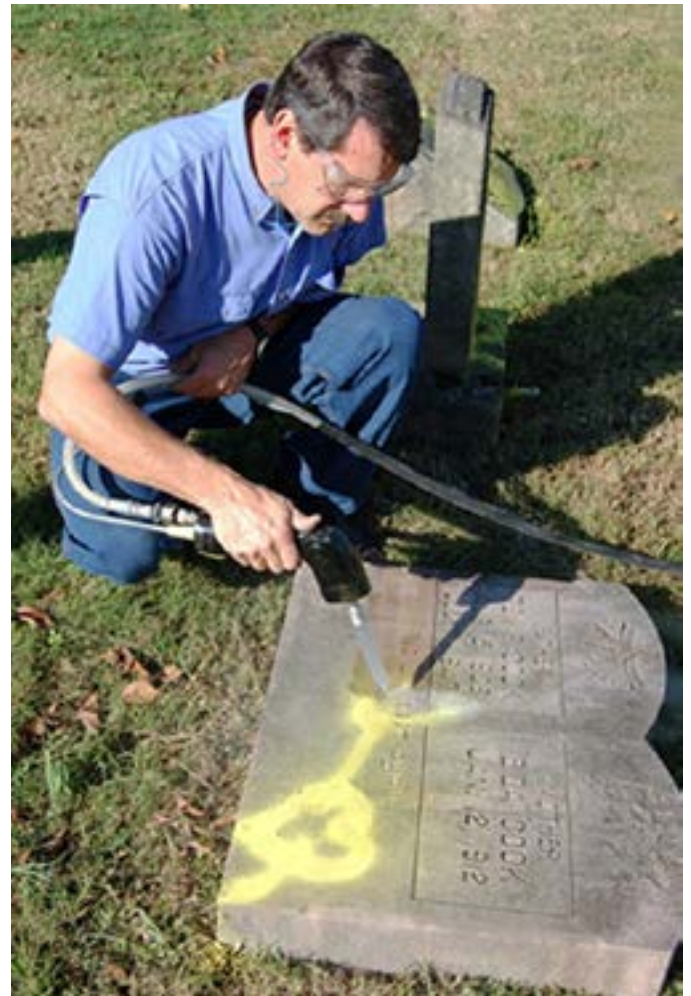
Figure 18. Graffiti is carefully removed using a low-pressure dry-ice misting instrument. Photo: Jason Church.
