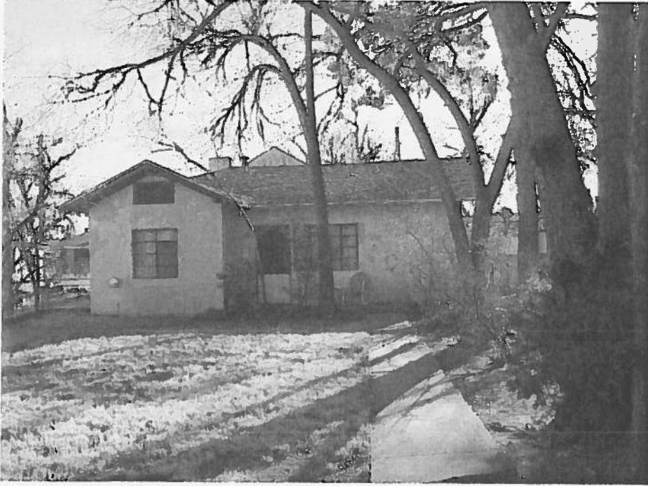
Figure 1: Subject property, 908 Roma Avenue NW.
