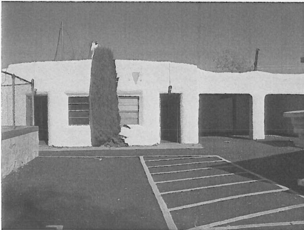
Aluminum replacement windows typical
