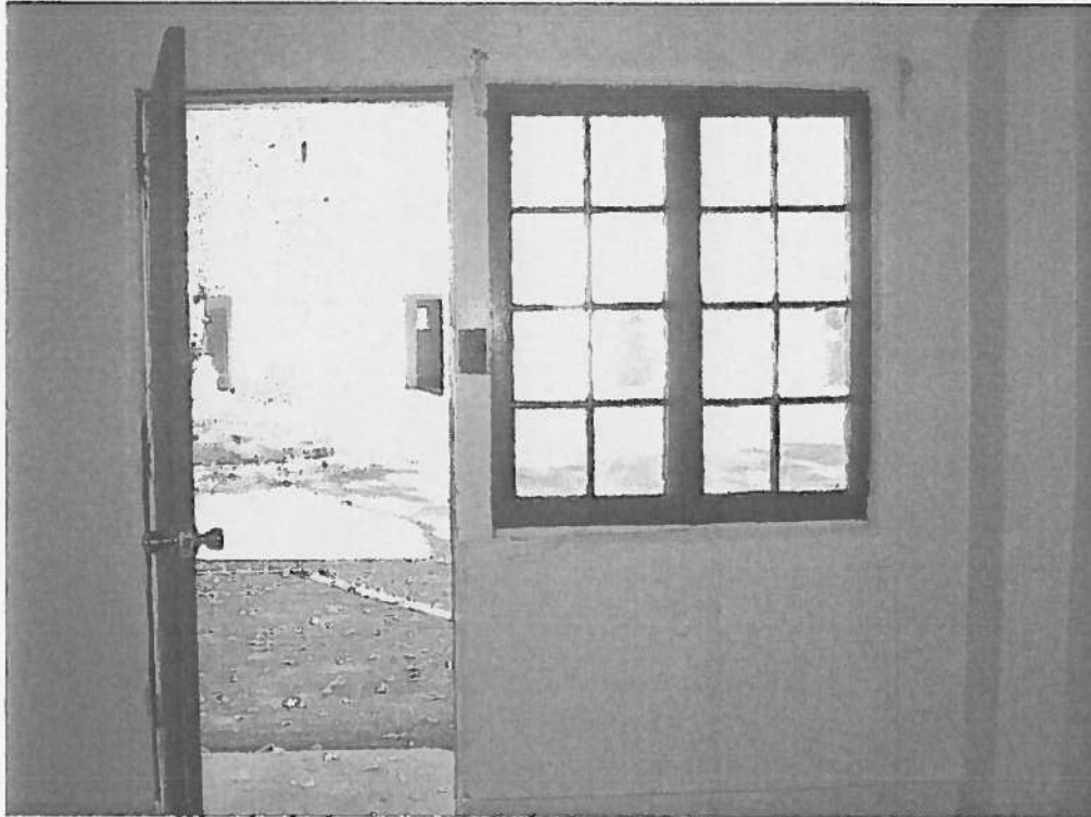
Wood windows were used where carports were enclosed
