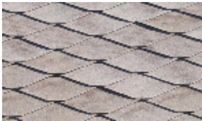
Asphalt shingles - This pattern was known as the "French method".
