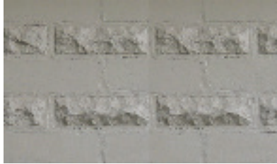
Mixed courses of cast stone and concrete blocks
