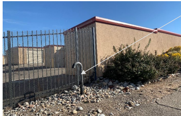
Existing landfill vent at adjacent self-storage facility
