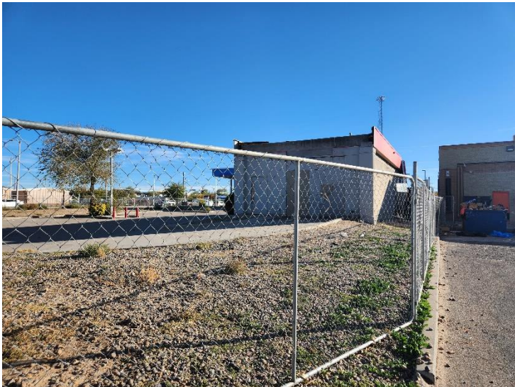
Figure 4: Viewing the northwestern portion of the subject site from Woodland Ave. NW. The former car wash can be seen from this direction.
