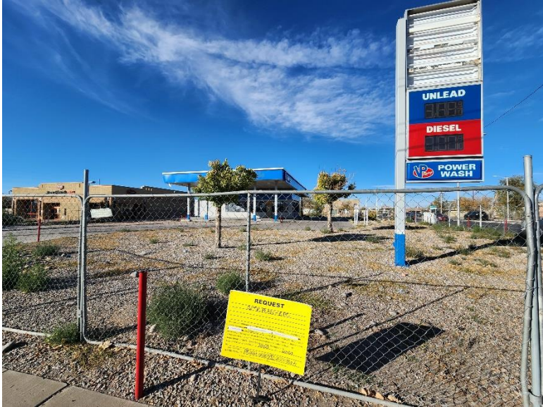
Figure 1: Looking north at the subject site from Menaul Blvd. The vacant gas station, convenient store and car wash can be seen. A sign posting is visible here.
