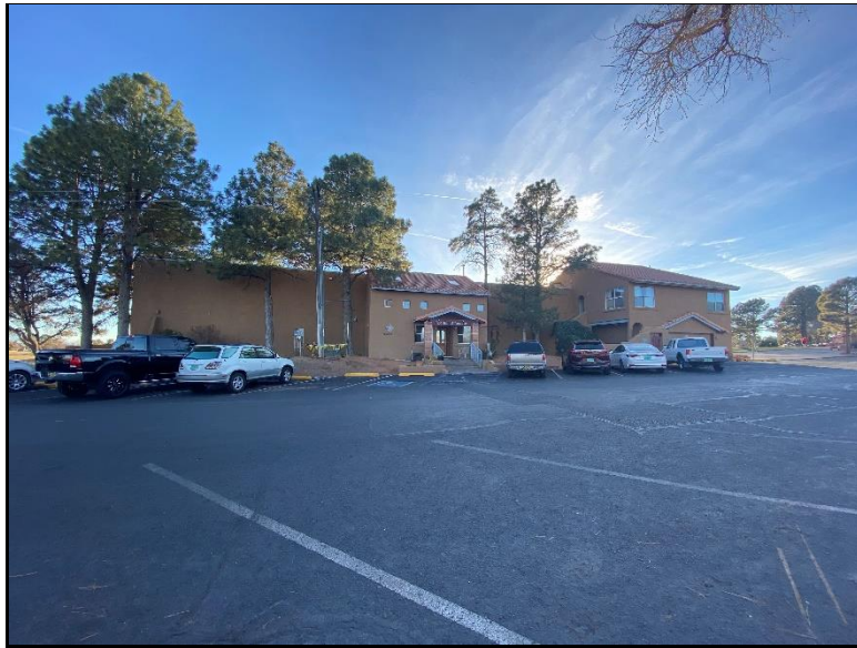
Figure 1: Looking south at the subject across Country Club Lane.
