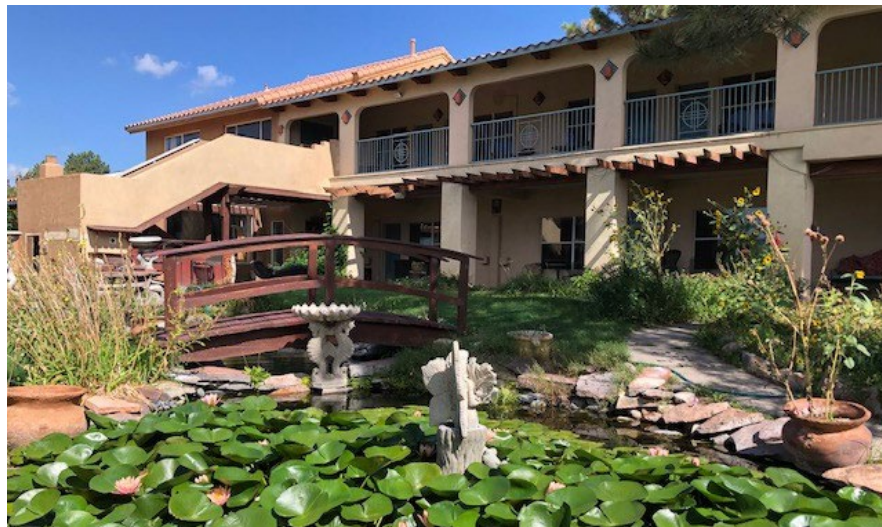
Private courtyard on the south side of the existing building.
