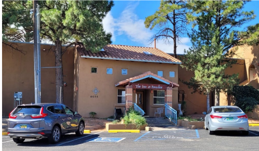
Entrance facing north to the existing building on the subject property.
