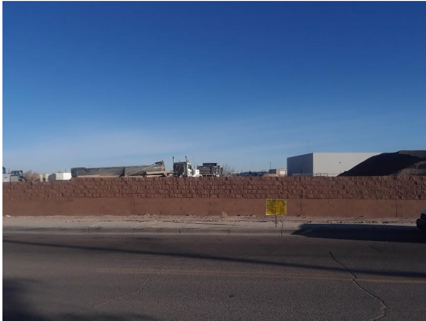
Figure 1: Looking N at Tract 4B, vacant lot for gravel loading into trucks.
