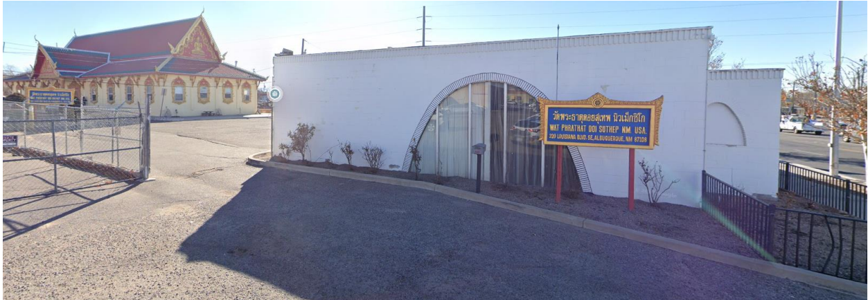
Figure 3: Looking SE at the existing building on the western portion of the subject site, which is proposed to be demolished and redeveloped.
