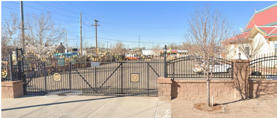
Figure 2: Looking west at the subject site from Alcazar St. at existing parking, fencing, and access.
