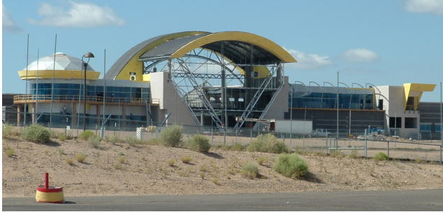
Balloon Museum under construction.
