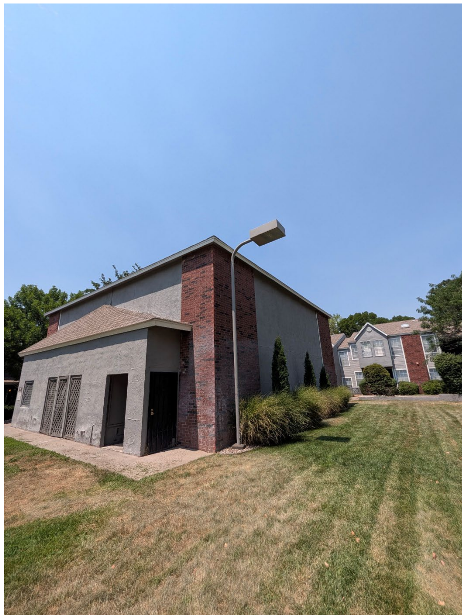
Figure 13: Northwest facing view of the former Racquetball Building (south and east façade) to be converted into 4, 2-story, studio dwelling units.
