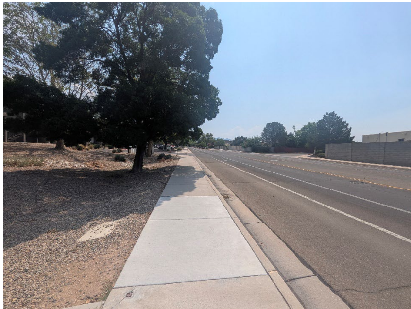
Figure 4 : South facing view from the far northwest corner of the subject site along Layton Ave. NE.
