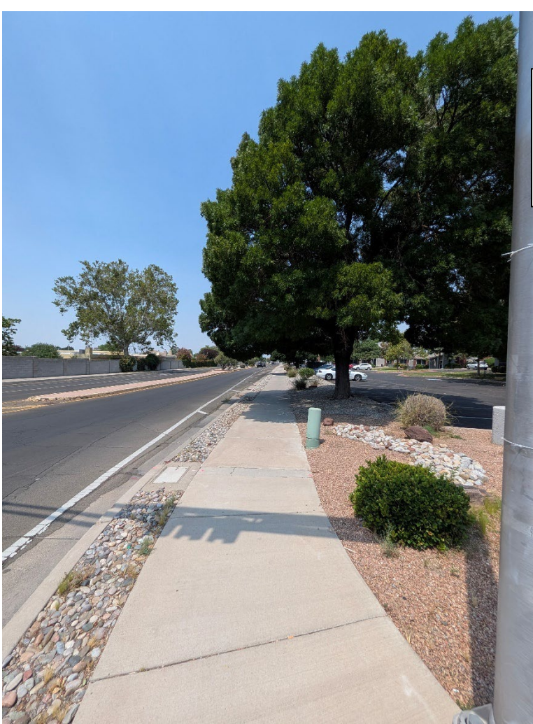
Figure 3 : Northwest facing view along Layton Ave NE. from the corner of Layton Ave. NE and Eubank Blvd. NE, the southernmost corner of the subject site.
