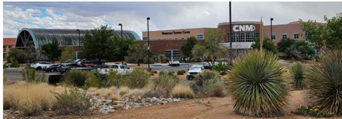
Caption: CNM Workforce Training Center North Entrance
