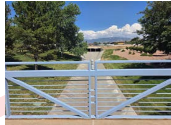
Caption: Pedestrian walkway over storm drain channel.
