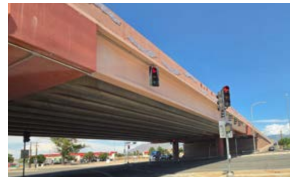
Caption: Paseo del Norte Boulevard at Osuna Road underpass
