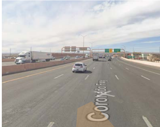
Caption: I-40 looking west
