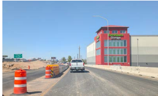
Caption: Southbound I-25 access road
