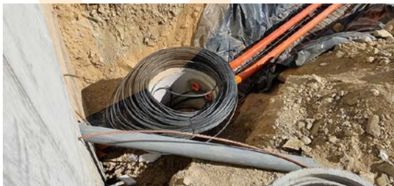
Caption: Fiber optic service installation.
