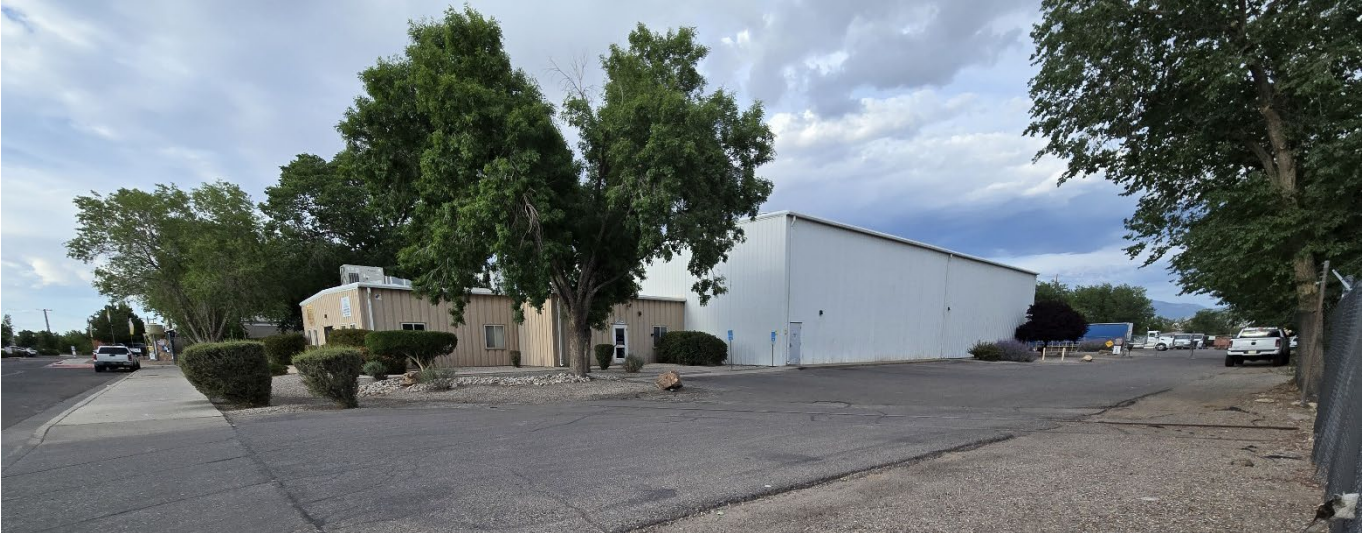
Figure 2: Overview of subject site - looking NE.
