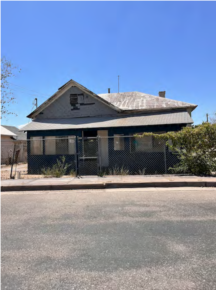
Photo of site frontage on Bellamah NW prior to fire.
