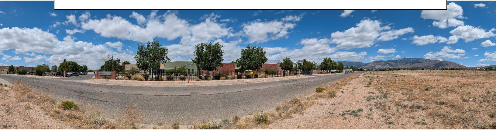
Figure 14 : NW facing panoramic view from across Stephen Moody St. SE with NMSBVI campus in view.
