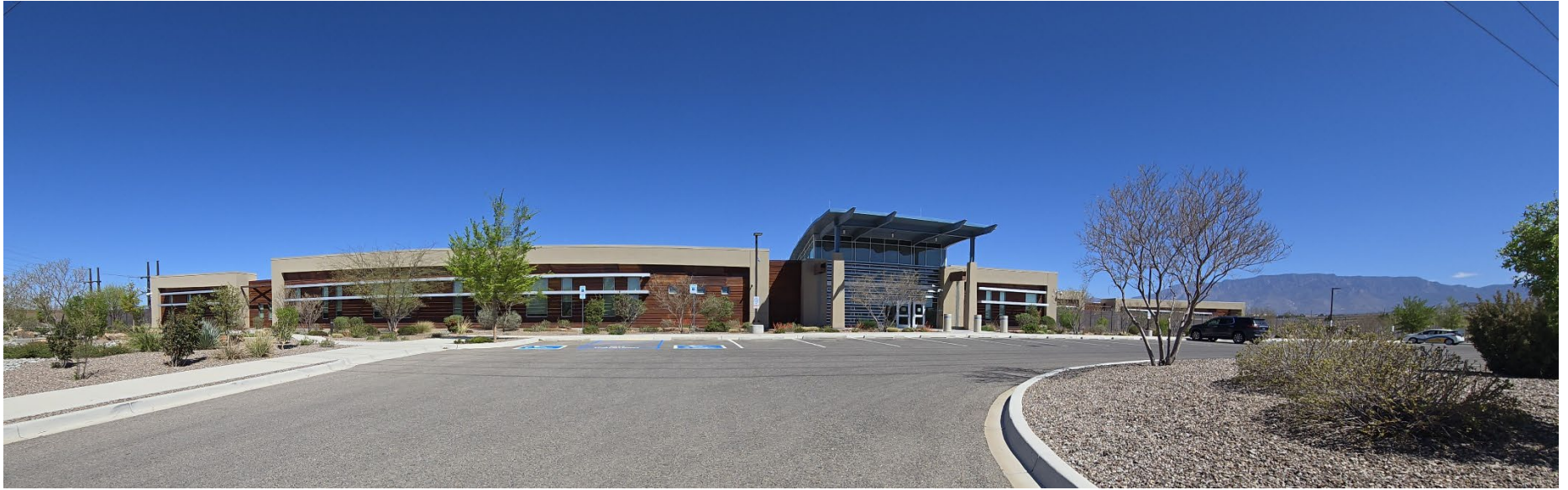
Figure 3: Overview of Customer Service building from Mission Ave. - looking ENE.
