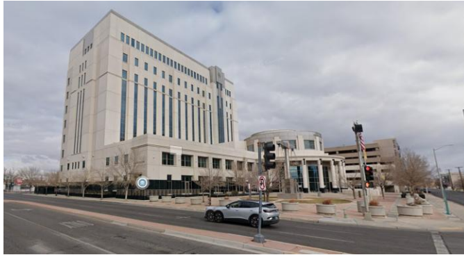
View of Bernalillo County Metropolitan Court and Parking Structure
