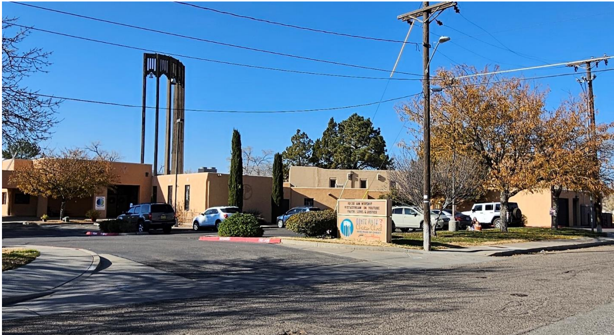
Figure 3: West facing subject site along Berkeley Pl. NE.
