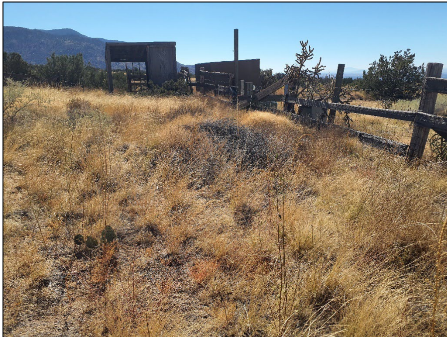
Figure 4. Survey area overview, wooden fenced area with recent building constructed of 2 x 6 lumber frame in the southwest corner, facing east (Frame -7324).
