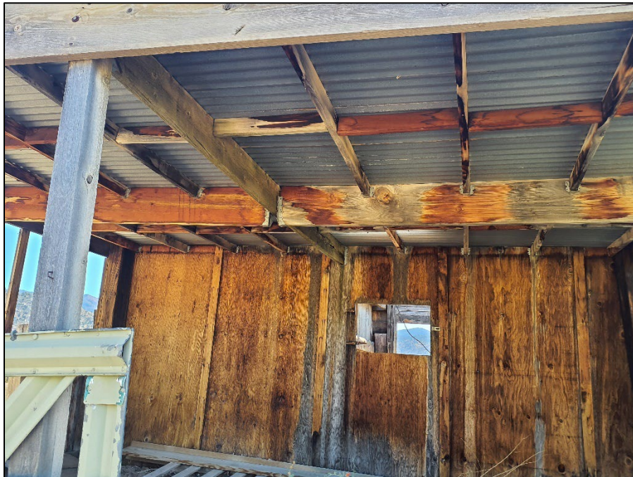
Figure 6. close-up showing modern construction, facing south (Frame -7075).
