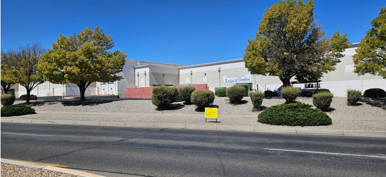
Pictures of Installed Signs, 9/4/24
