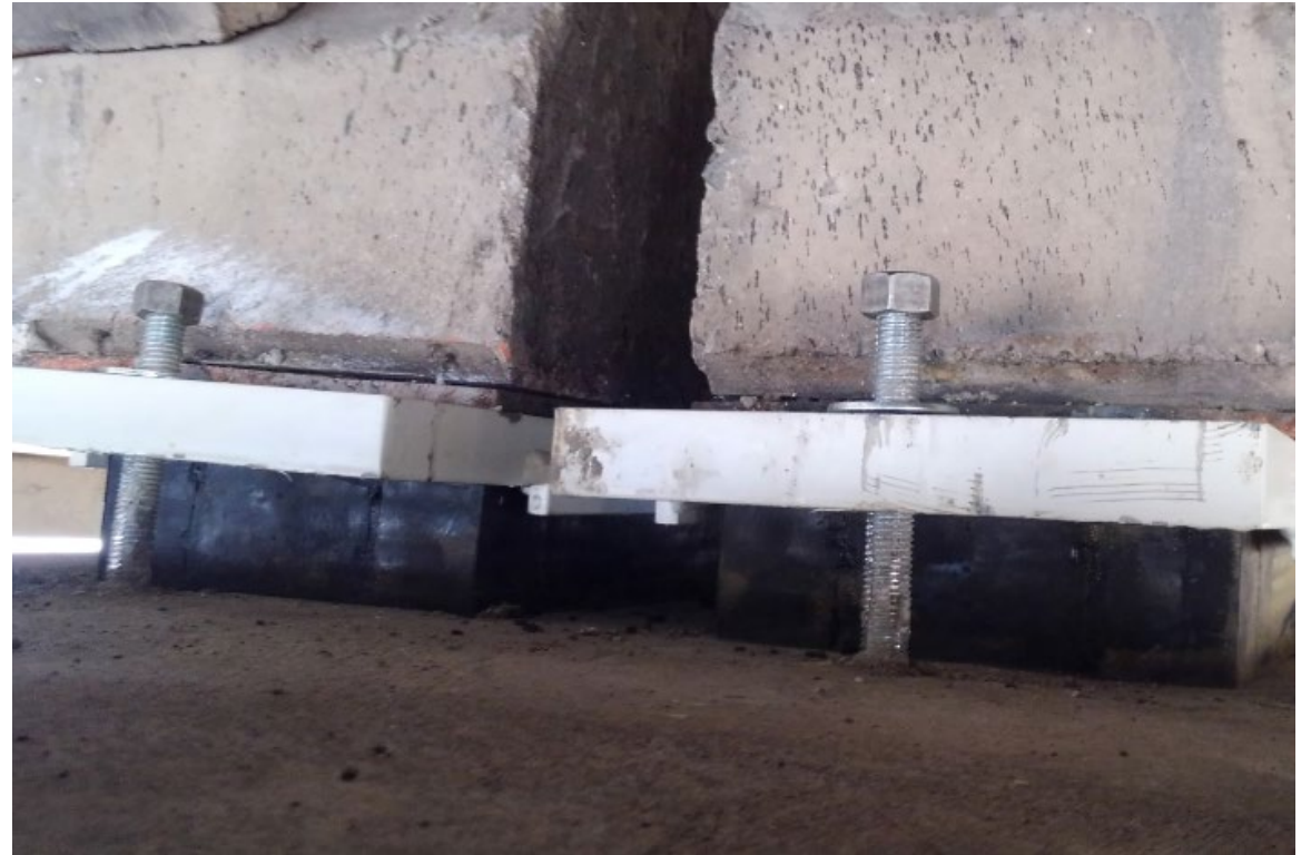
Emergency Repair (After)
