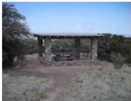
30 & 31. Foothills Shade Structures
