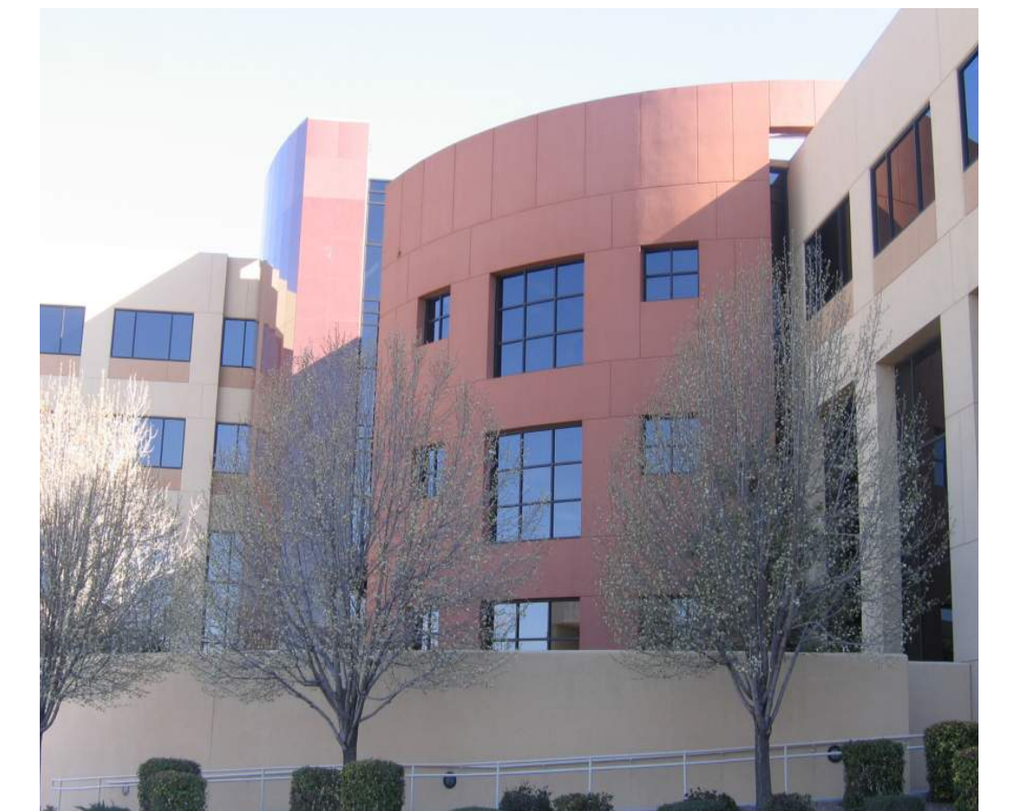
Altura Office Building
