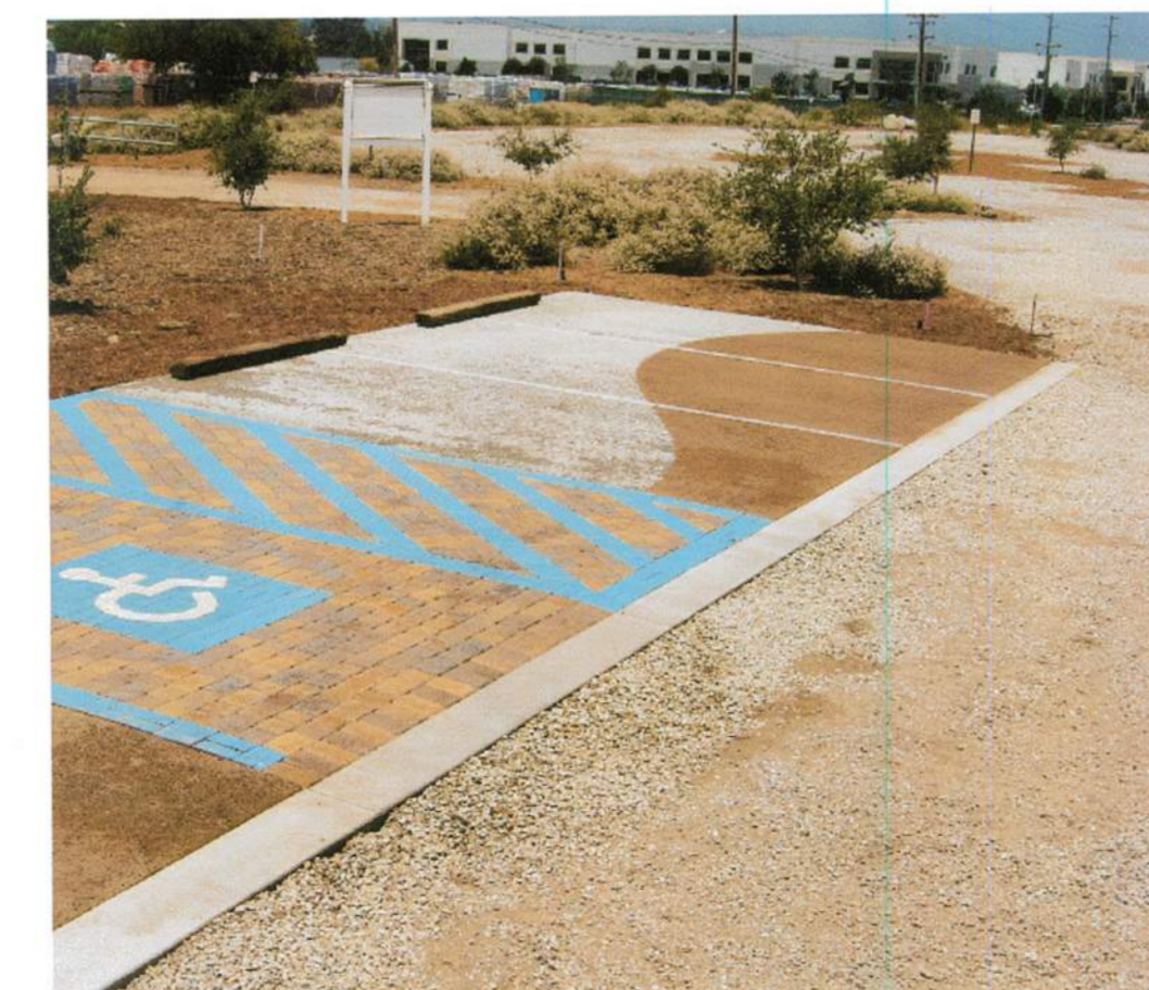
Pervious Surface Materials on Parking Lot
