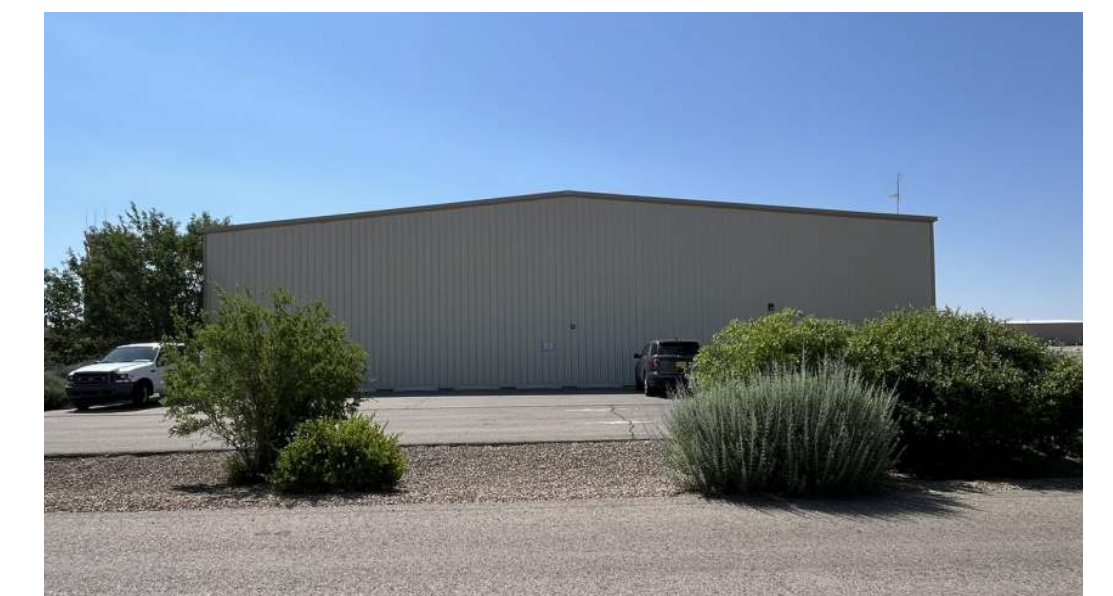
Existing Stormwater Control from an Executive Hangar
