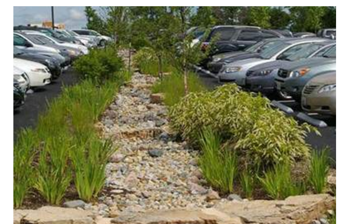
Parking Island Stormwater Control Area
