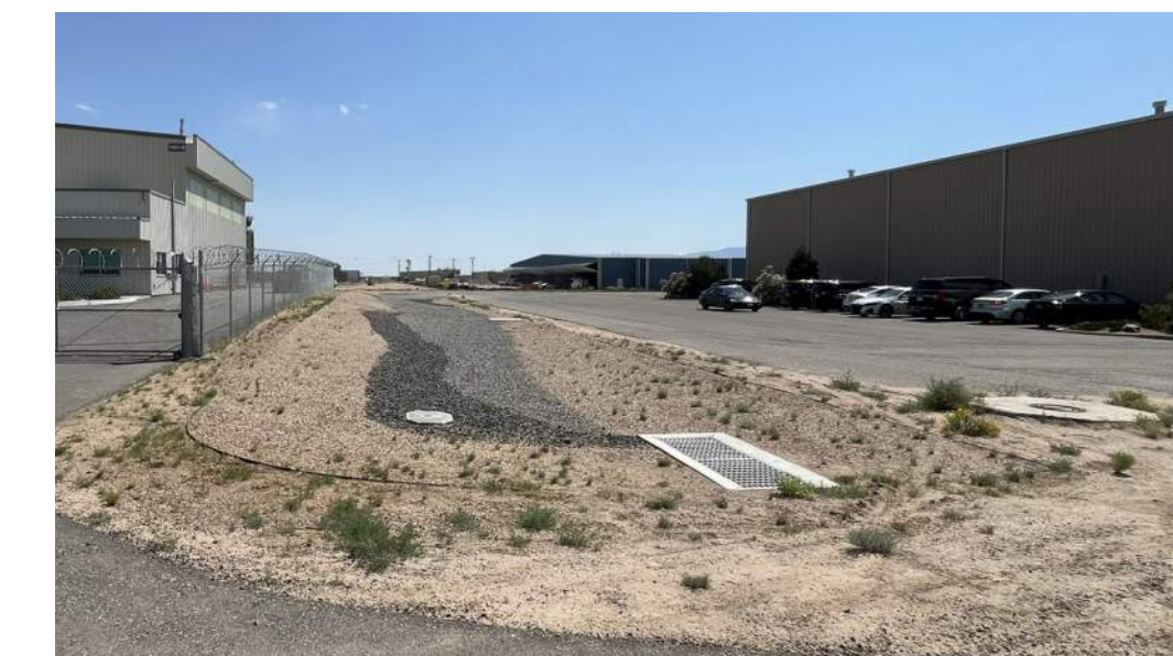
Existing Stormwater Control at NM State Police Hangar
