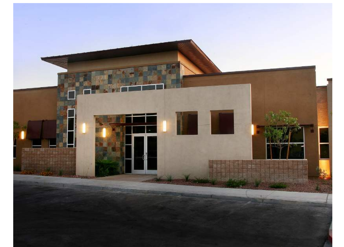
Red Rock Office Building
