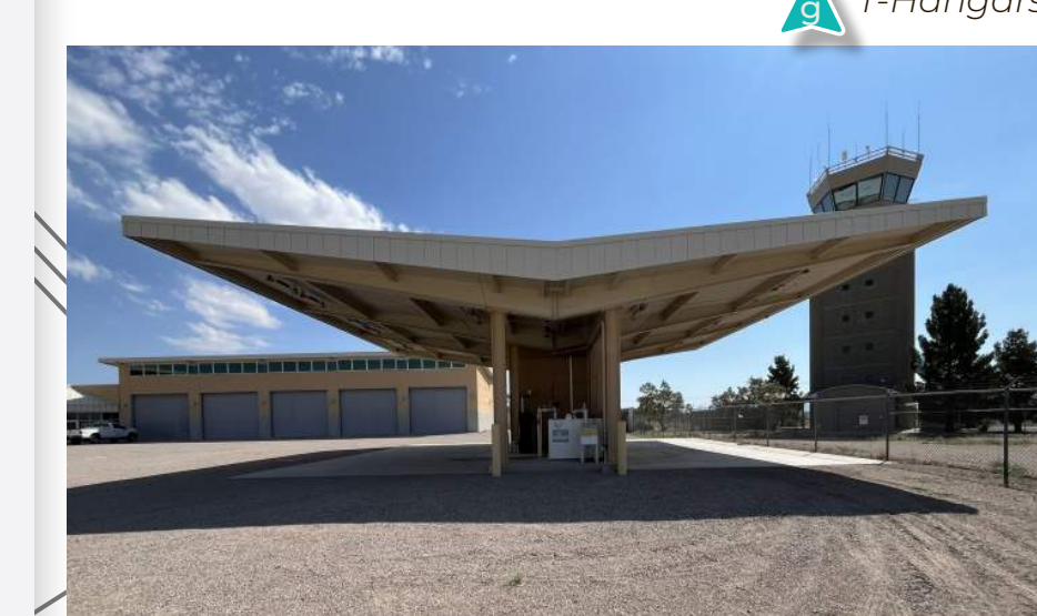
Vehicle Fueling Facility
