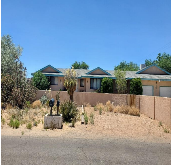
Front of 4815 Northern Trail NW – Looking West
