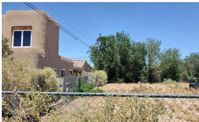
View of a portion of 4815 Northern Trail NW from Westward LN NW
