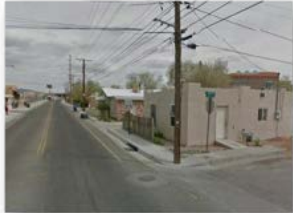
Photo 4. Utility Pole Within Curb Ramp
