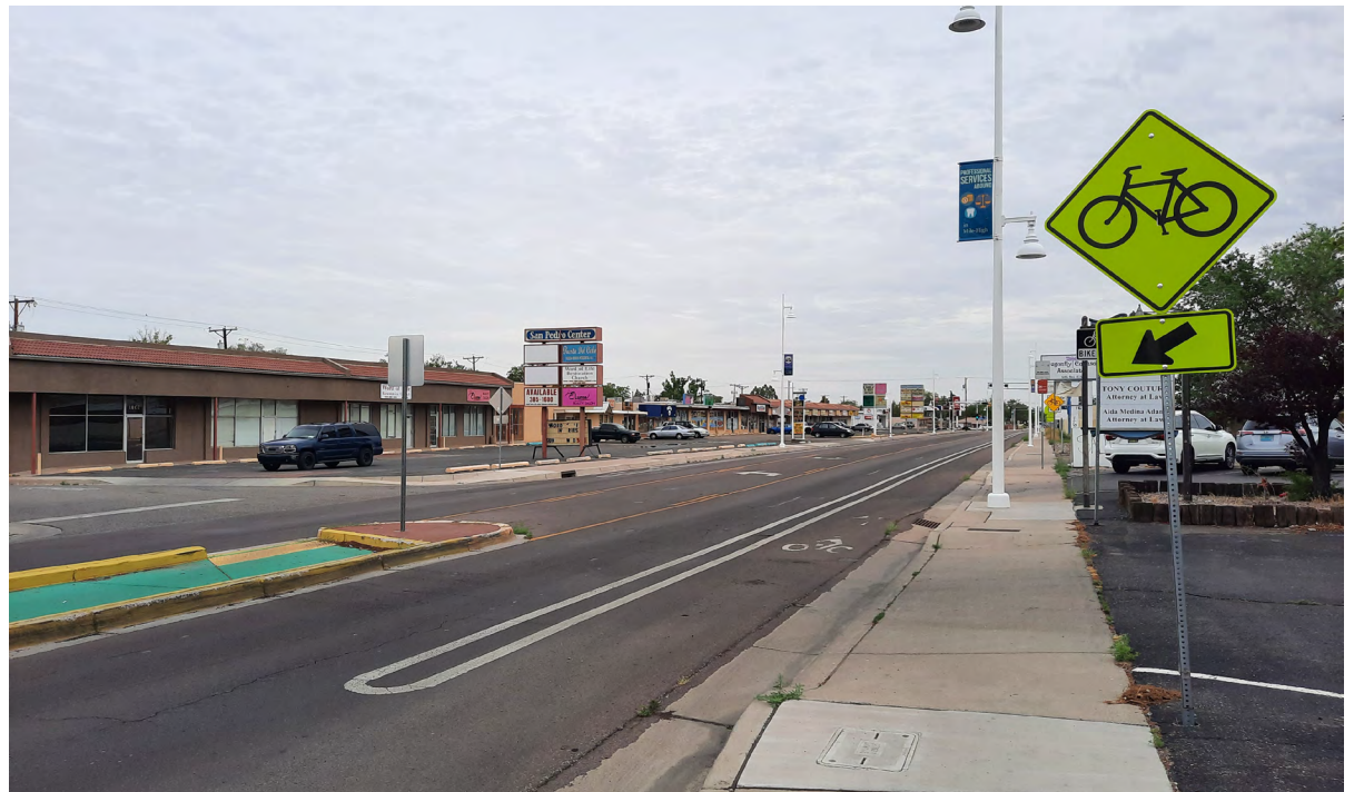
The City installed buffered bike lanes along San Pedro Drive as part of a road diet in which one lane of traffic was removed in each direction to reduce travel speeds and create safer conditions for people walking and biking.
