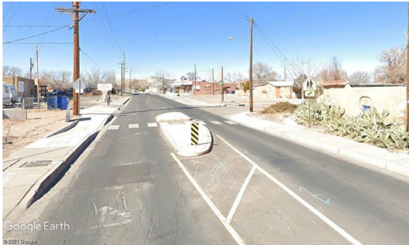
Figure 5: High Visibility Crosswalk Markings and Signage on Mountain Rd
