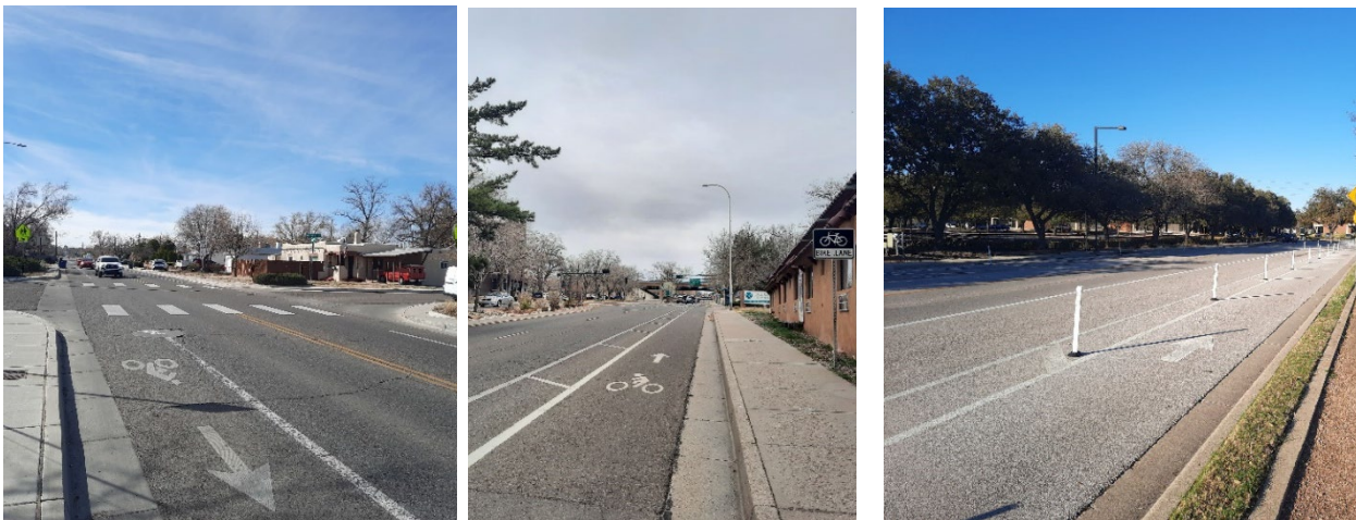
Figure 14. Bike Lane Facilities: Standard Bike Lane (Left), Buffered Bike Lane (Center), and Separated Bike Lane (Right)
