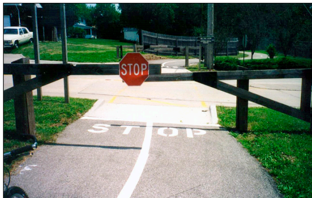
Figure 5-21: Gates across a bicycle path (not recommended)
