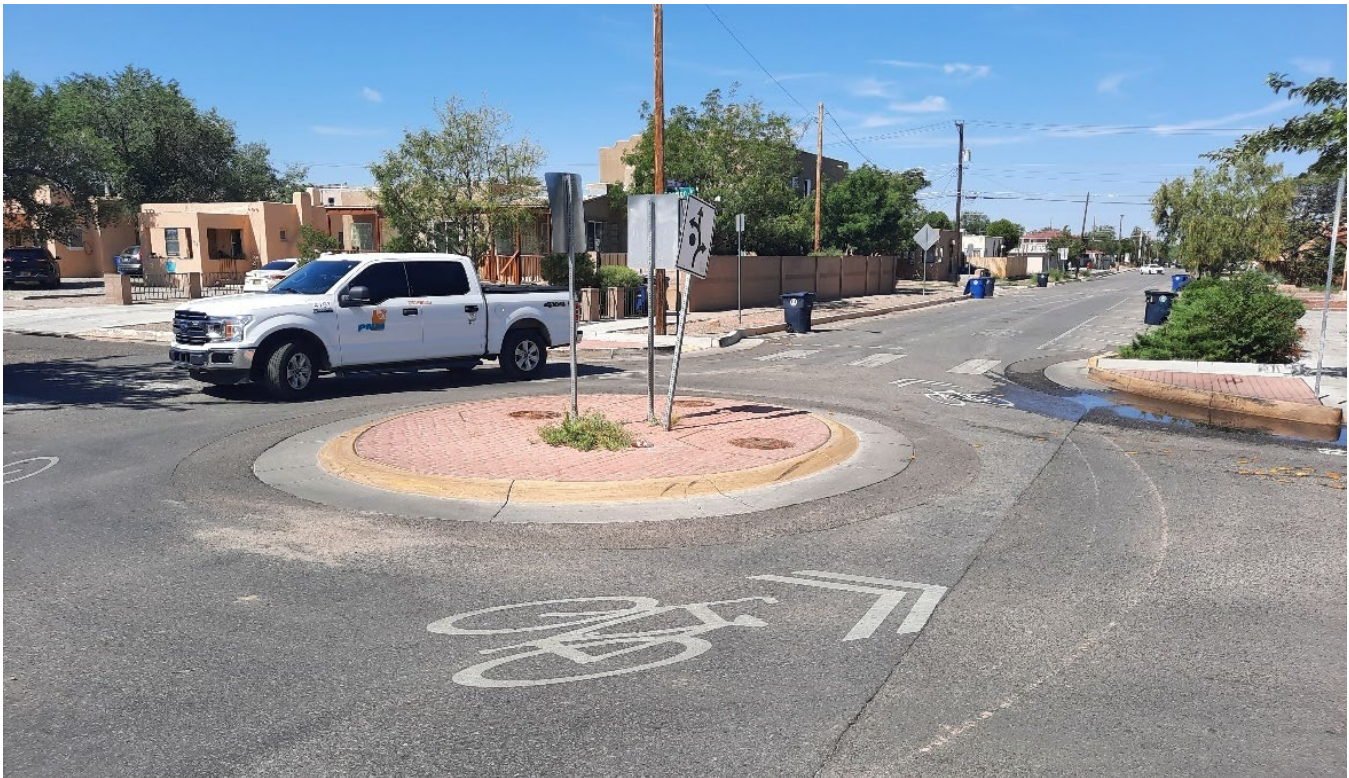
Figure 19: Mini Traffic Circle along Silver Ave Bike Boulevard
