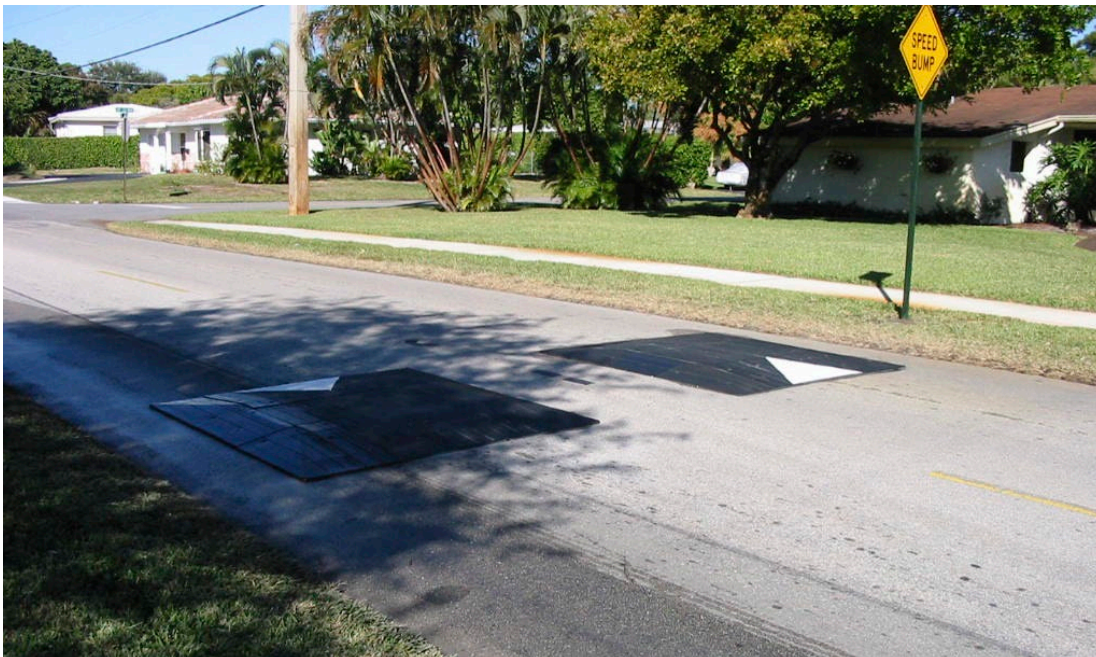
Figure 21: Example of Speed Cushion
