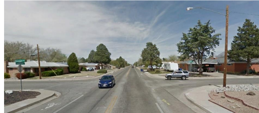
Figure 53: Existing Crossing at Pennsylvania St
