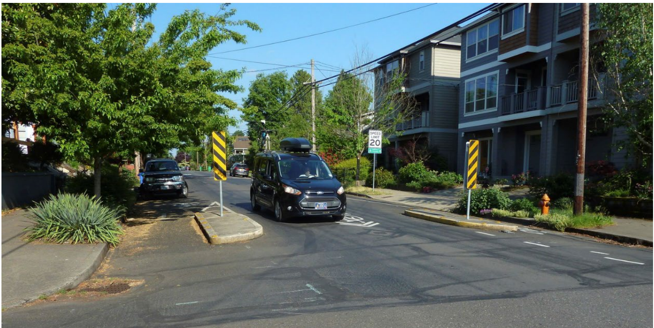
Figure 17: Example of One Lane Pinch Point
