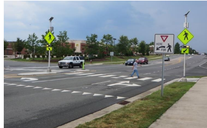
Figure 16: Rectangular Rapid Flashing Beacon on Multi-Lane Arterial
