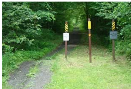
Photo of bollards on the Delaware and Hudson Rail Trail in Pawlet VT. Trail users created a new trail to get around the bollards. Photo by Jon Kaplan, Bicycle and Pedestrian Program Manager, Vermont Agency of Transportation.
