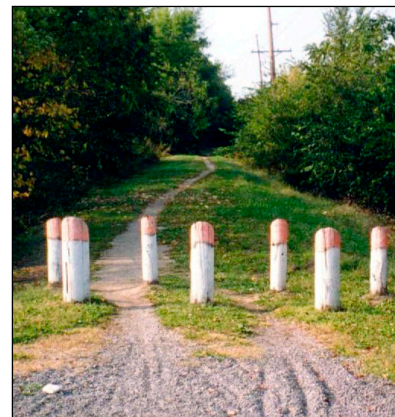
Too many bollards inhibit path access.
