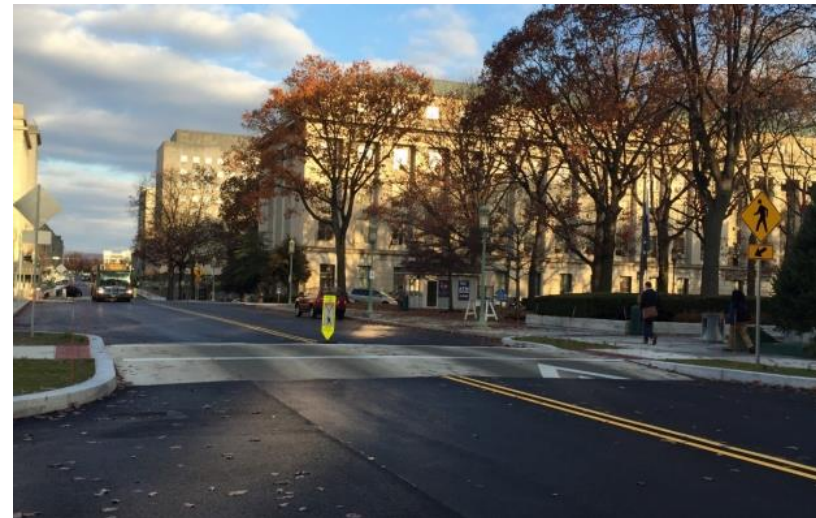
Figure 25: Raised Crosswalk with Curb Extension and In-Street Pedestrian Crossing Sign
