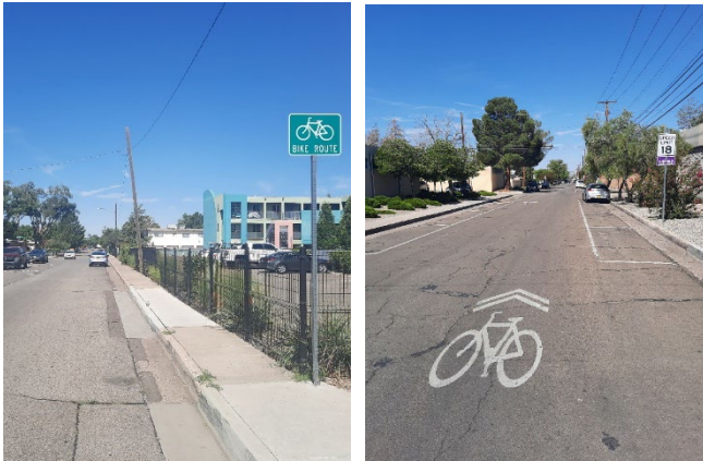
Figure 13. Shared Street Facilities: Bike Route (left) and Bike Boulevard (right)
