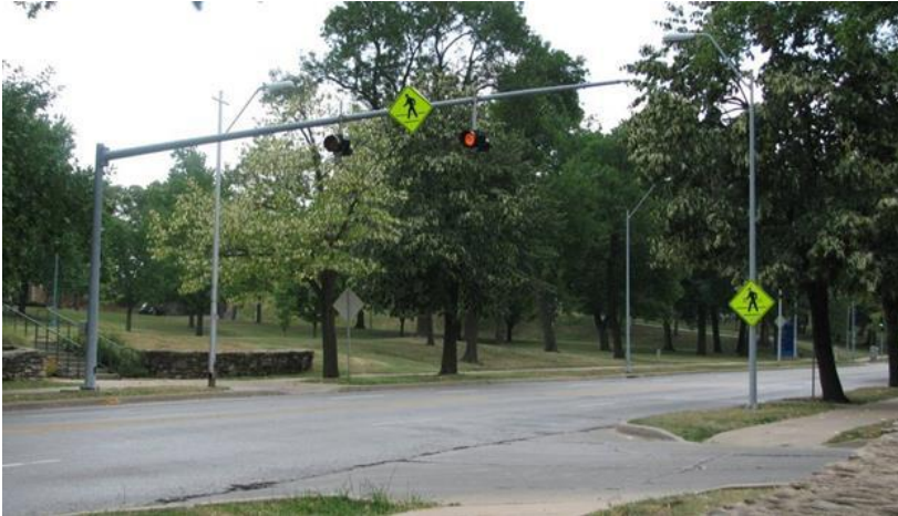
Figure 14: Overhead Flashing Lights Example
