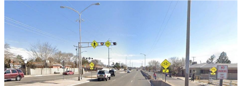
Figure 47: Existing Trail Crossing at Wyoming Blvd
