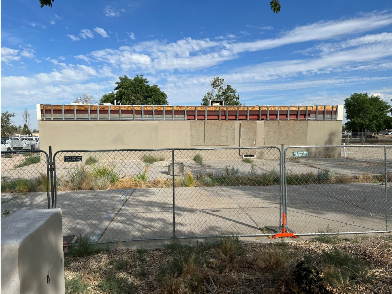
Figure 7: East Side of subject site
