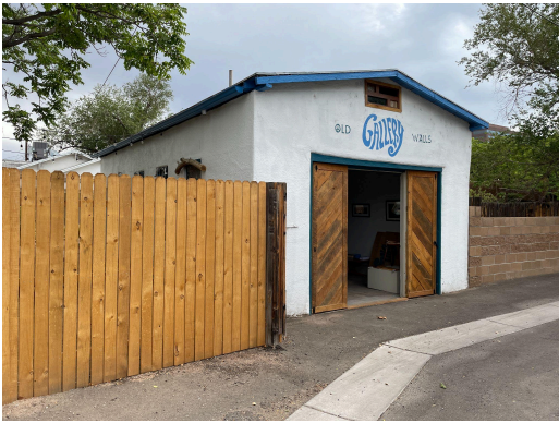
Image 1: Old Walls Gallery (exterior)
