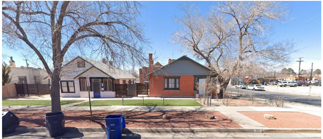
View looking west to the subject property
