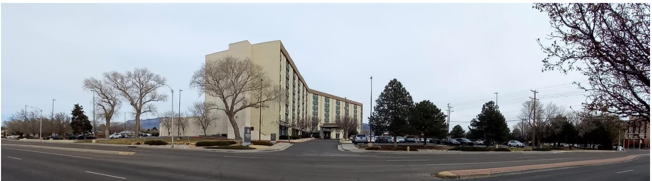
Figure 5: Panoramic overview of the subject site looking east.
