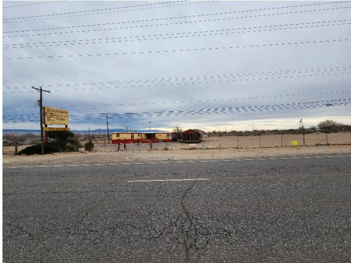
Viewing the subject site from Central Ave SW. A sign posting can be seen in this view and old manufactured homes left by a previous manufactured home retailer.
