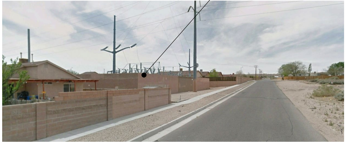
View looking west along Sunset Gardens, with the subject property on the right. A pair of high voltage circuits is also visible in the photo – these lines run by the western side of the subject property.
