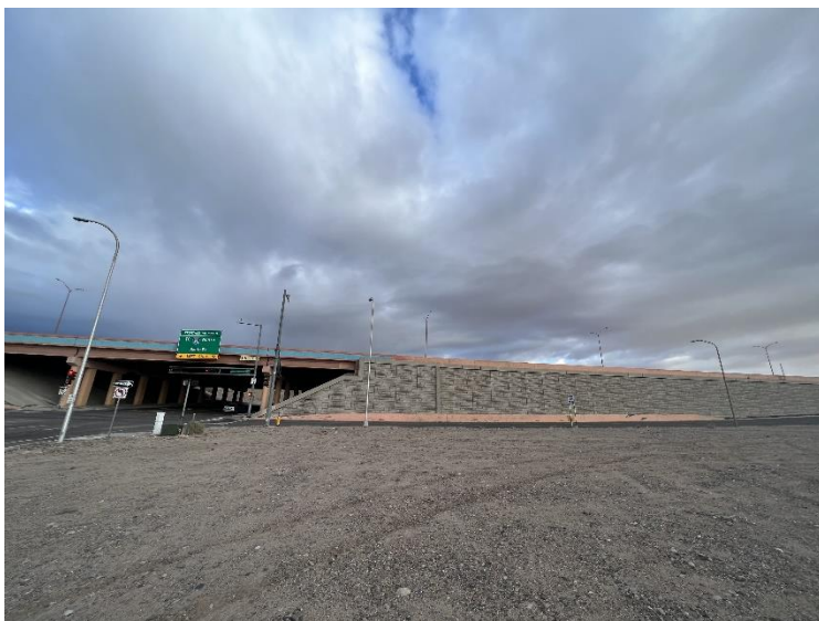
Figure 6: Looking east of the subject site towards I-25 and Frontage Rd. S.
