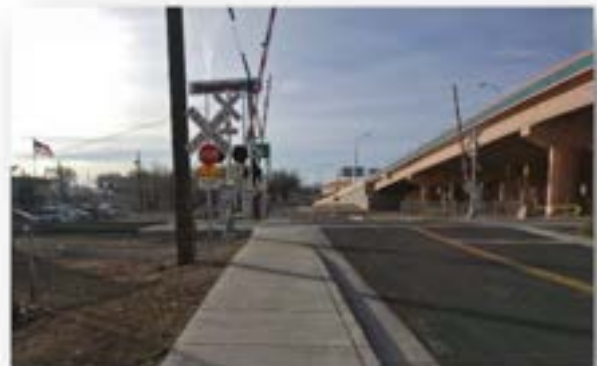
Photo 1. Looking west at RR crossing on Indian School
