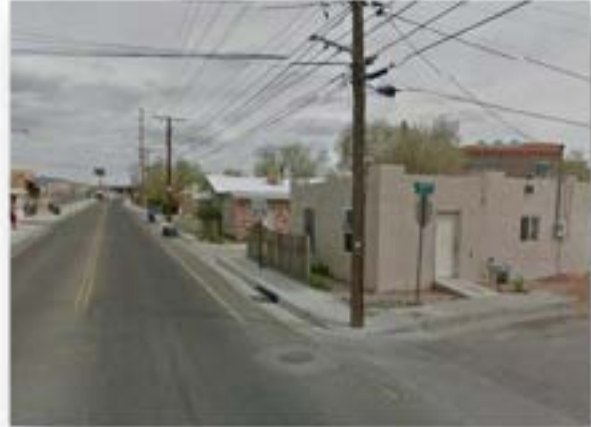
Photo 4. Utility Pole Within Curb Ramp
