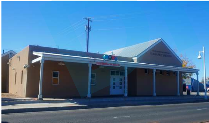
Caption: Old Town Police Substation
