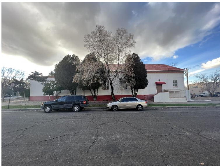
Figure 4: Looking west towards a property zoned R-ML, which currently appears to feature commercial and/or institutional uses.
