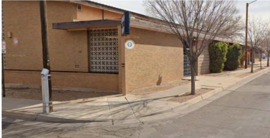
Figure 2 Street View of Subject Site
