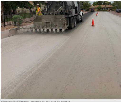
Treating pavement in Phoenix. COURTESY OF THE CITY OF PHOENIX
