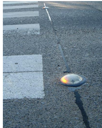
FIGURE 4-11 Example of Grade-Level Caution Lights
