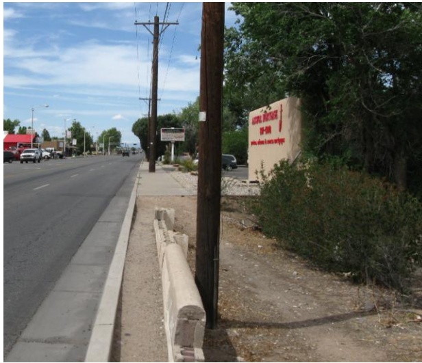
FIGURE 4-7 Unpaved and Obstructed Sidewalk
