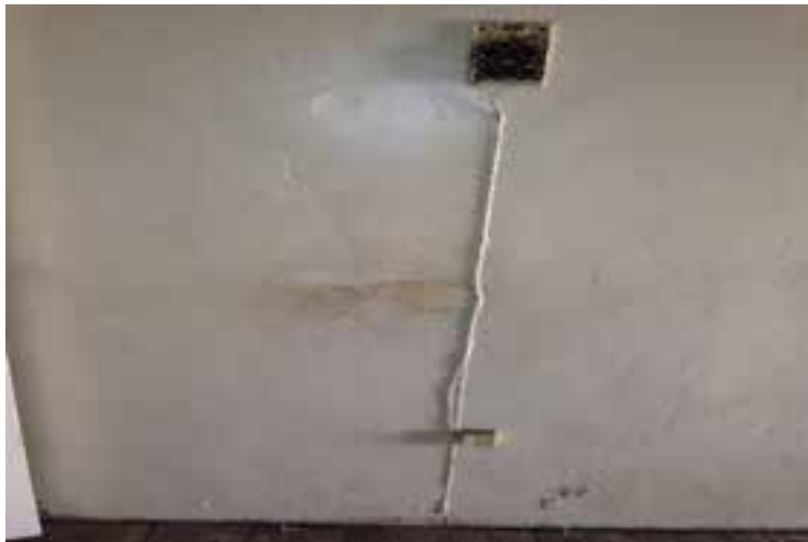
Guest Room Telephone Line and Telephone Jack Connector
