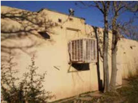
Added Building 'A' Evaporative Cooler
