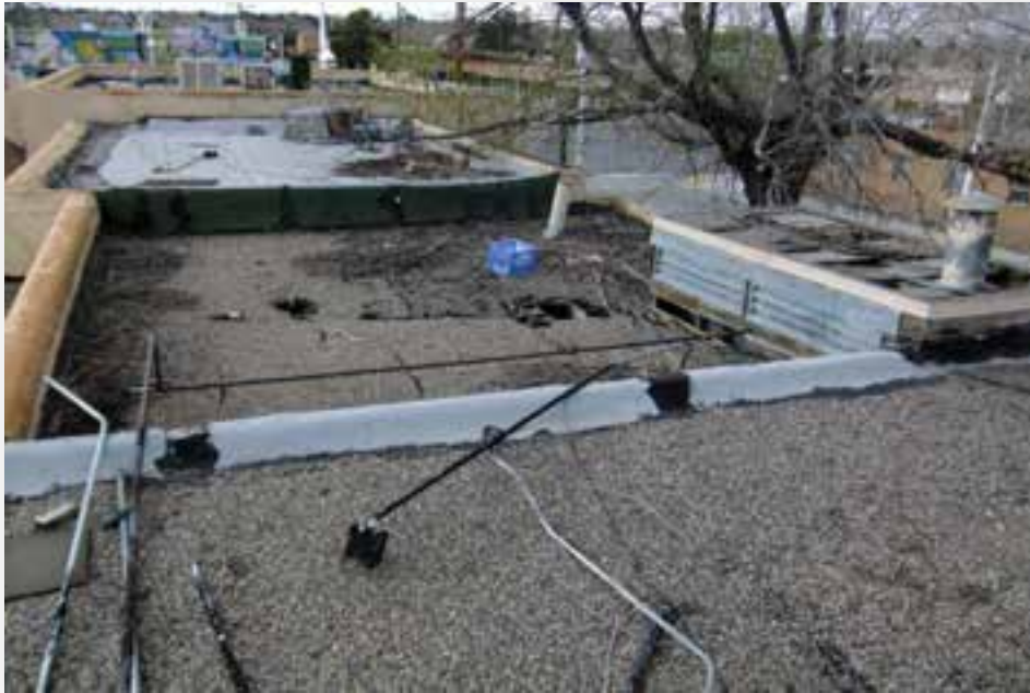
Figure 46- Building G Roof Failure
