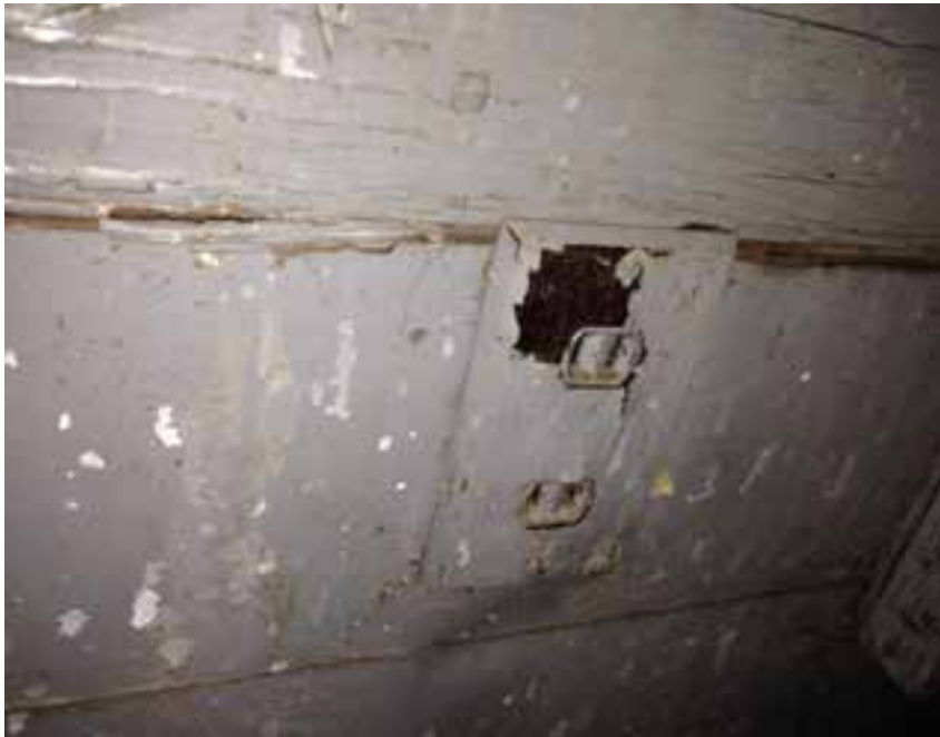
Non-Grounded Receptacle Through-out the Facility-Bldg's A, B, C, D, E, F & G
