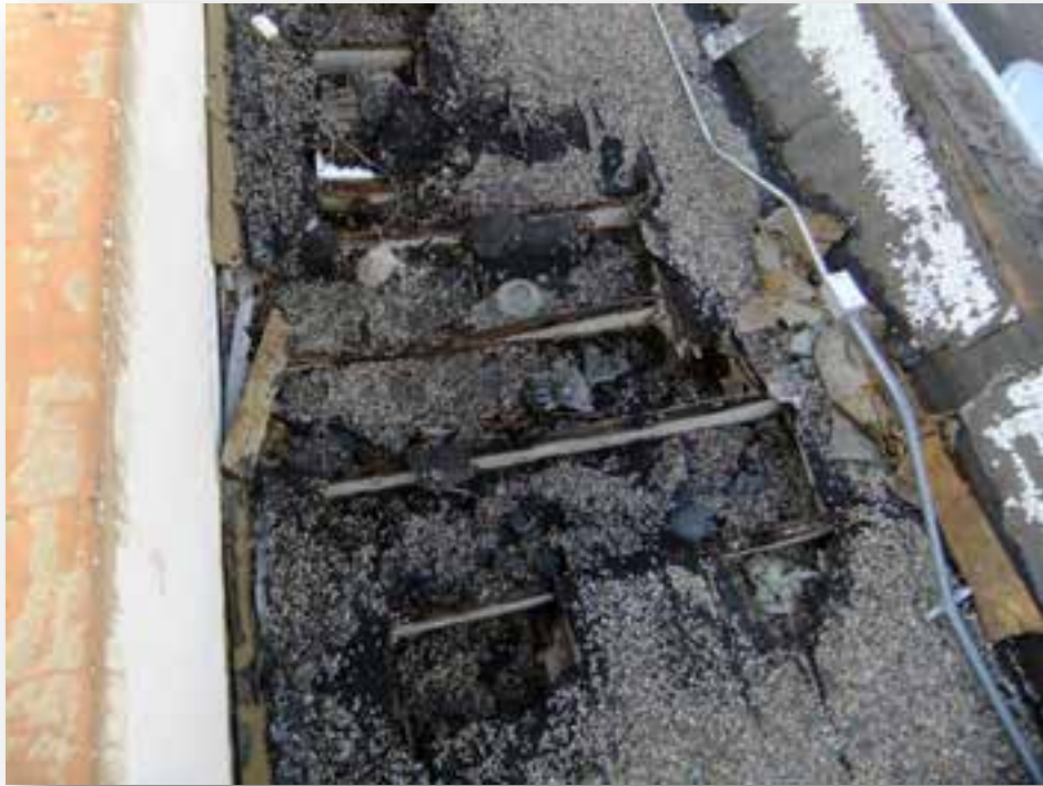
Figure 1 - Building A Roof
