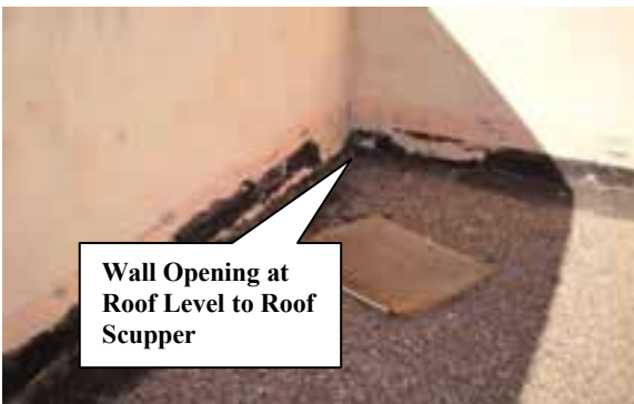
Roof Drainage Lobby West End
