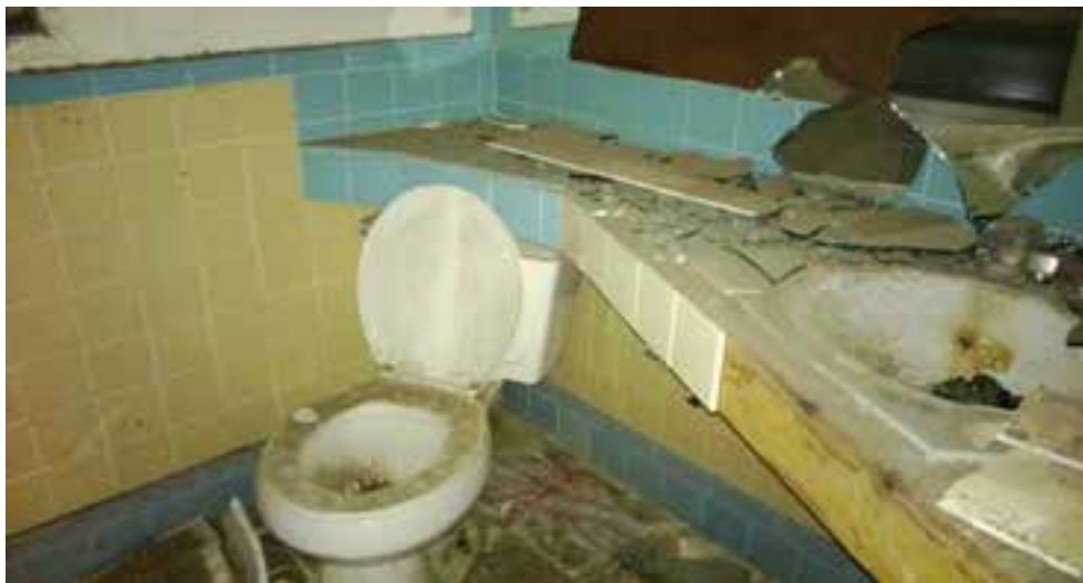
Water Closet and Lavatory
