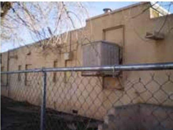
Added Building 'G' Evaporative Cooler
