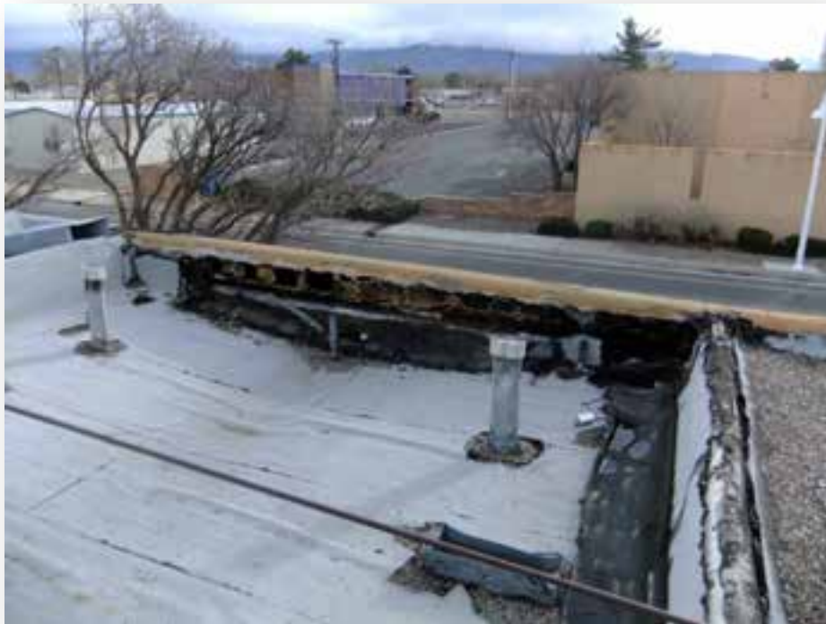
Figure 9- Building B Roof Deterioration at Partial Collapse
