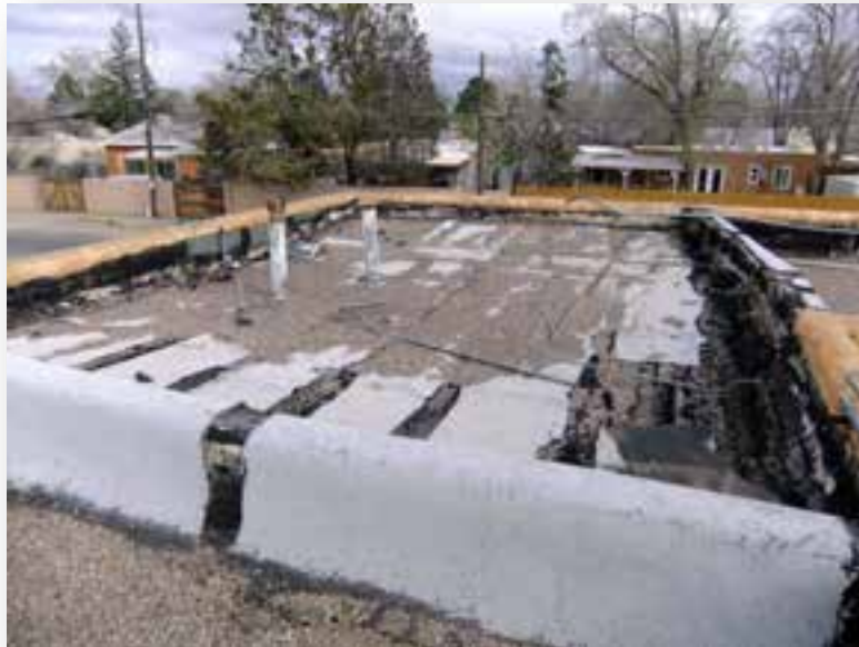
Figure 38- Building F Roof – Missing Flashing
