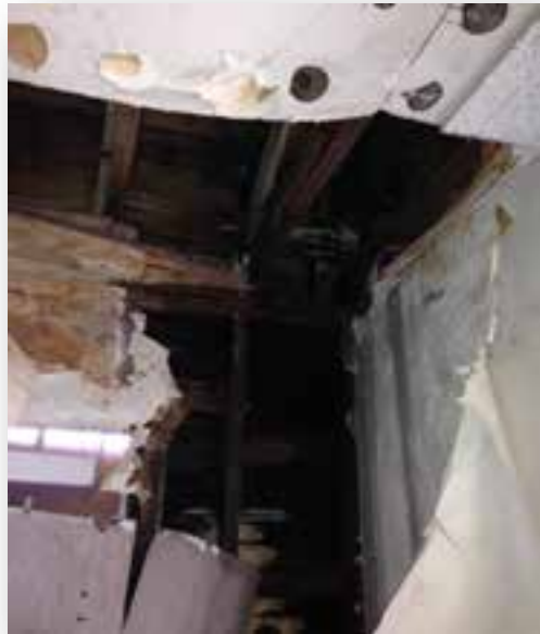
Figure 36- Building E 2 nd Floor Water Infiltration
