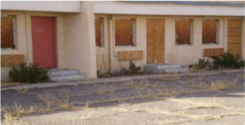
PTAC units with Plywood Cover
