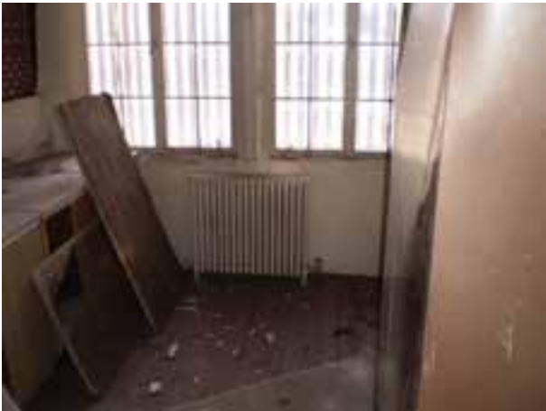
Room Steam Radiator – Manual Control
