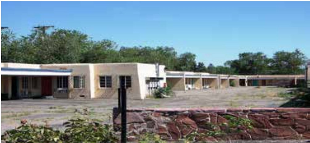
Undated Photo Showing PTAC units installed
