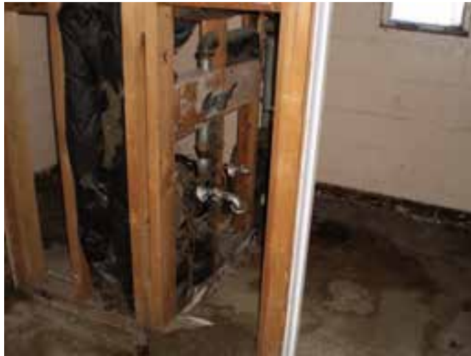
Missing Plumbing Fixtures, Water Closet and Lavatory
