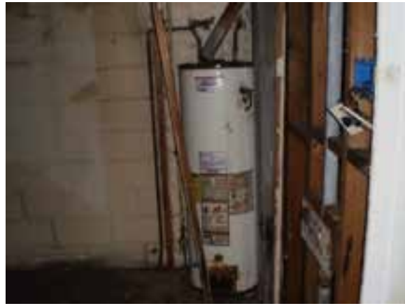
Natural Gas Kitchen Domestic Water Heater
