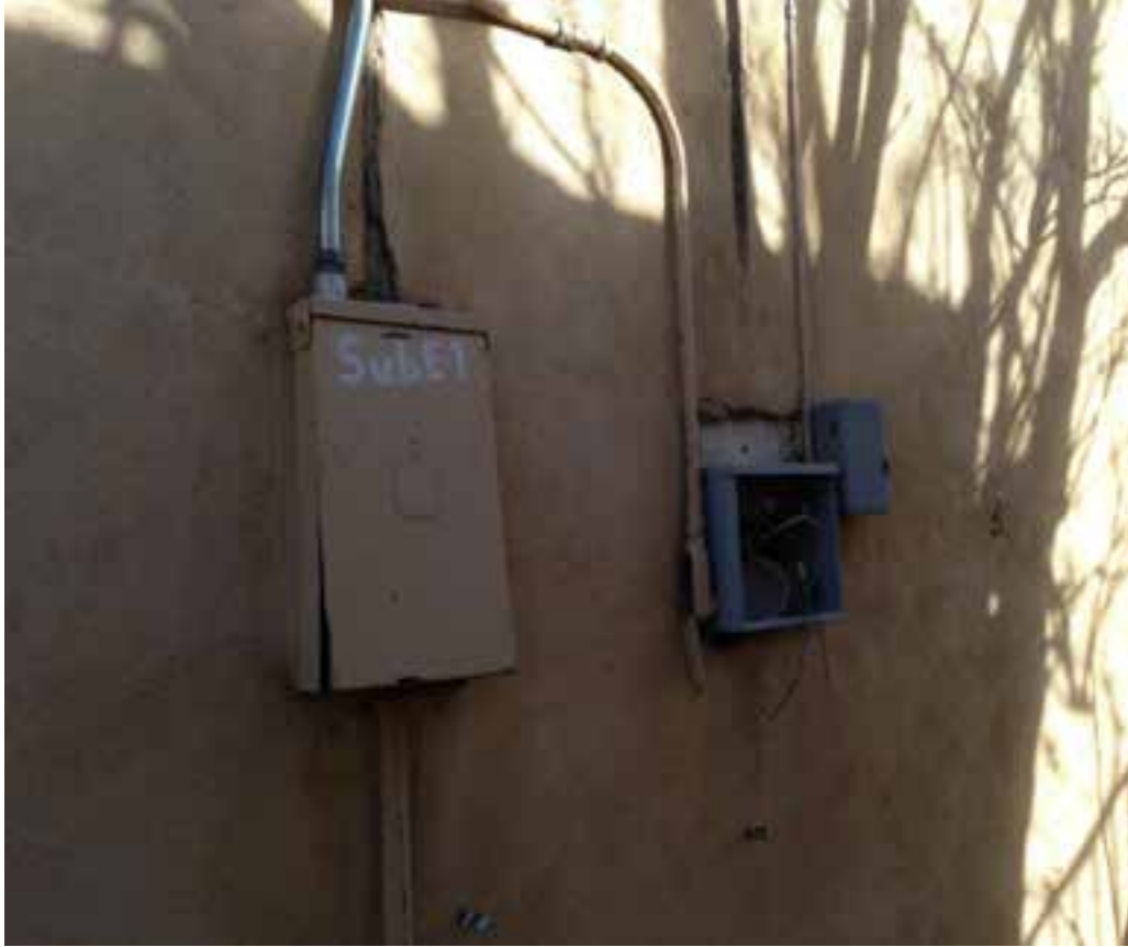
Building “B”– Sub Panel “E1” Mounted On The South Exterior Wall Of Bldg. “B”
