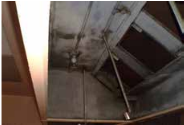
Kitchen Range Hood Fire Protection
