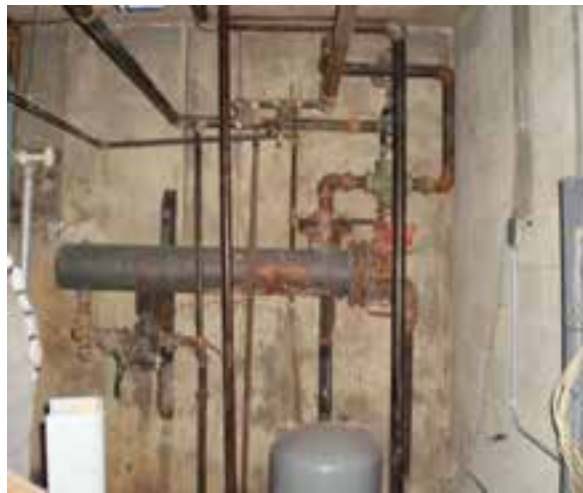
Steam To Hot Water Heat Exchanger
