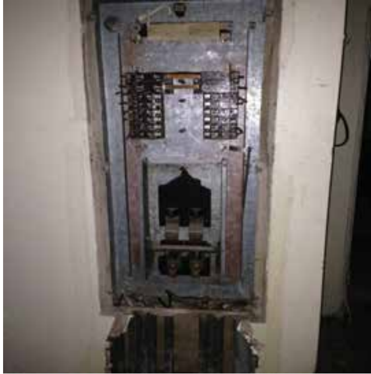
Sub-Panel Located In Hall Of Office Building "E"
