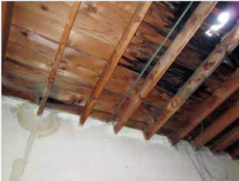
Figure 4- Building A Room 103 – Roof Deterioration
