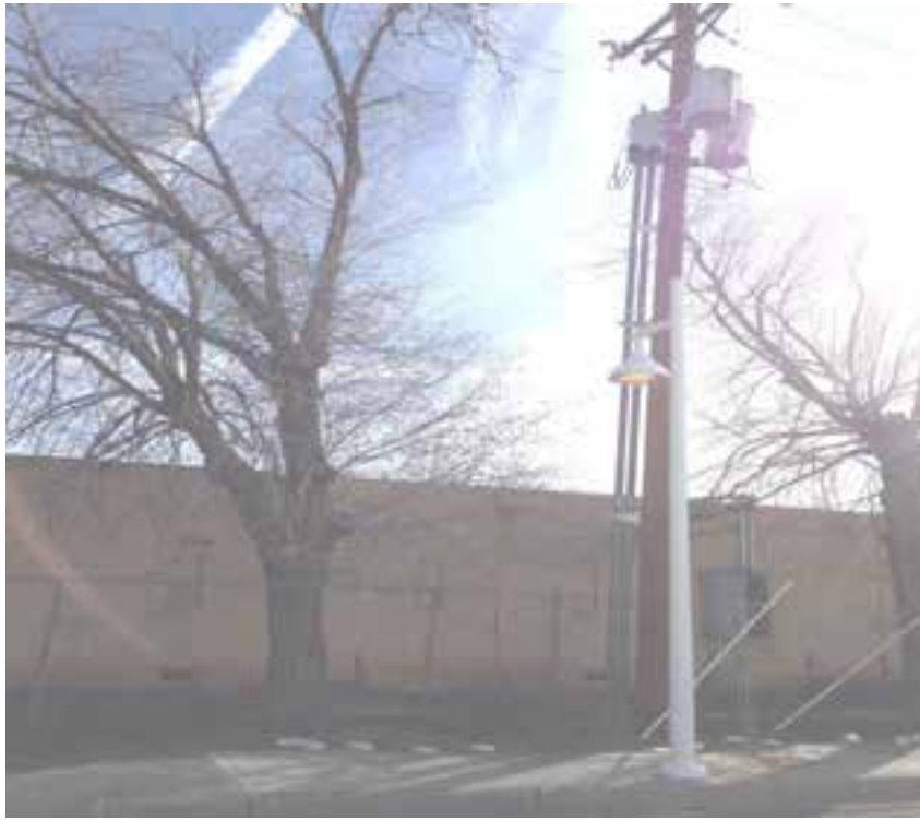
PNM Service Riser to Meter/Can Equipment – Exterior West Building “G”
