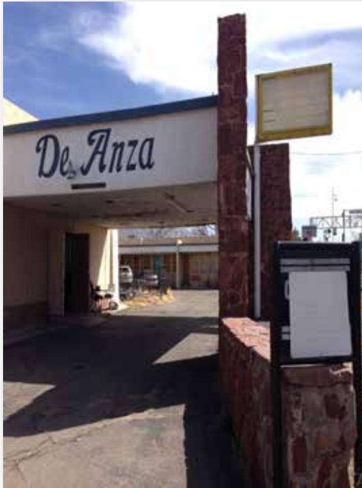
Figure 37- Building E Porte Cochere
