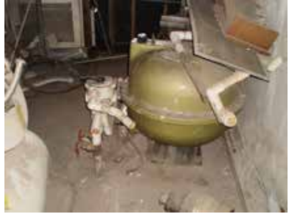
Swimming Pool Support Equipment
