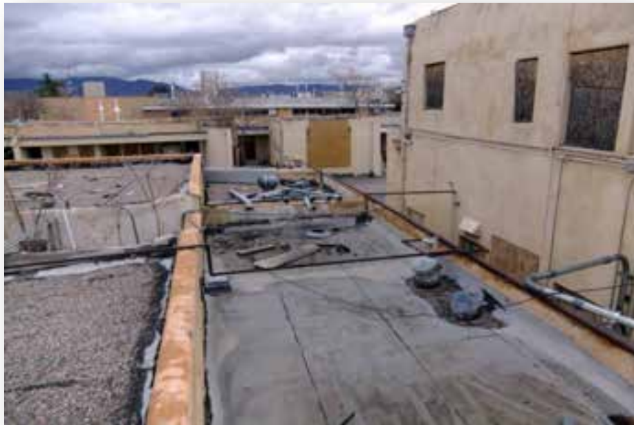
Figure 27-Building D Roof Damage
