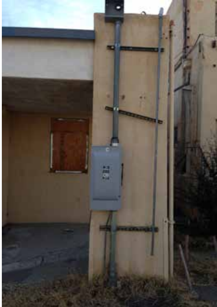
Disconnect Switch Located At West Exterior Wall Building “D”
