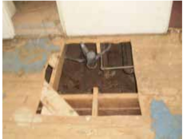
Plumbing Piping Below Floor in Typical Room
