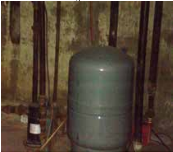
Steam Condensate Pump
