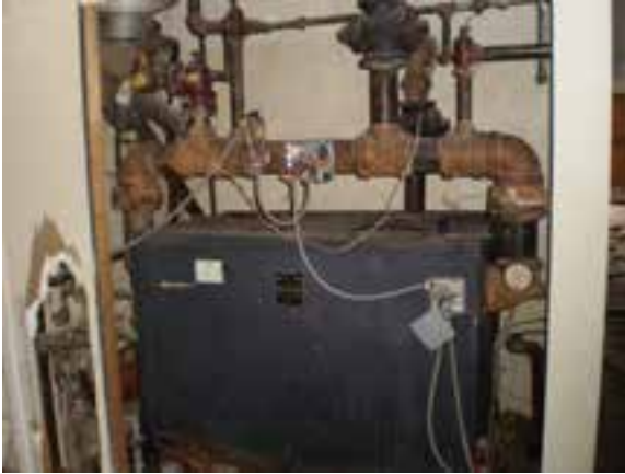
Swimming Pool Natural Gas Boiler
