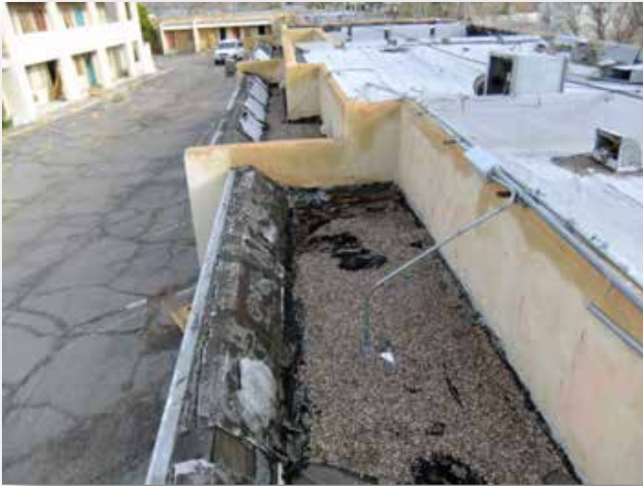
Figure 8- Building B Roof Deterioration on West Canopy
