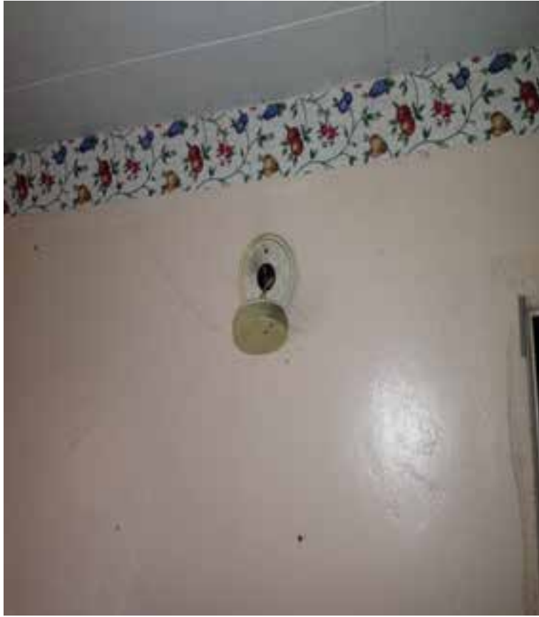
Guest Room Fire Alarm Smoke Detector
