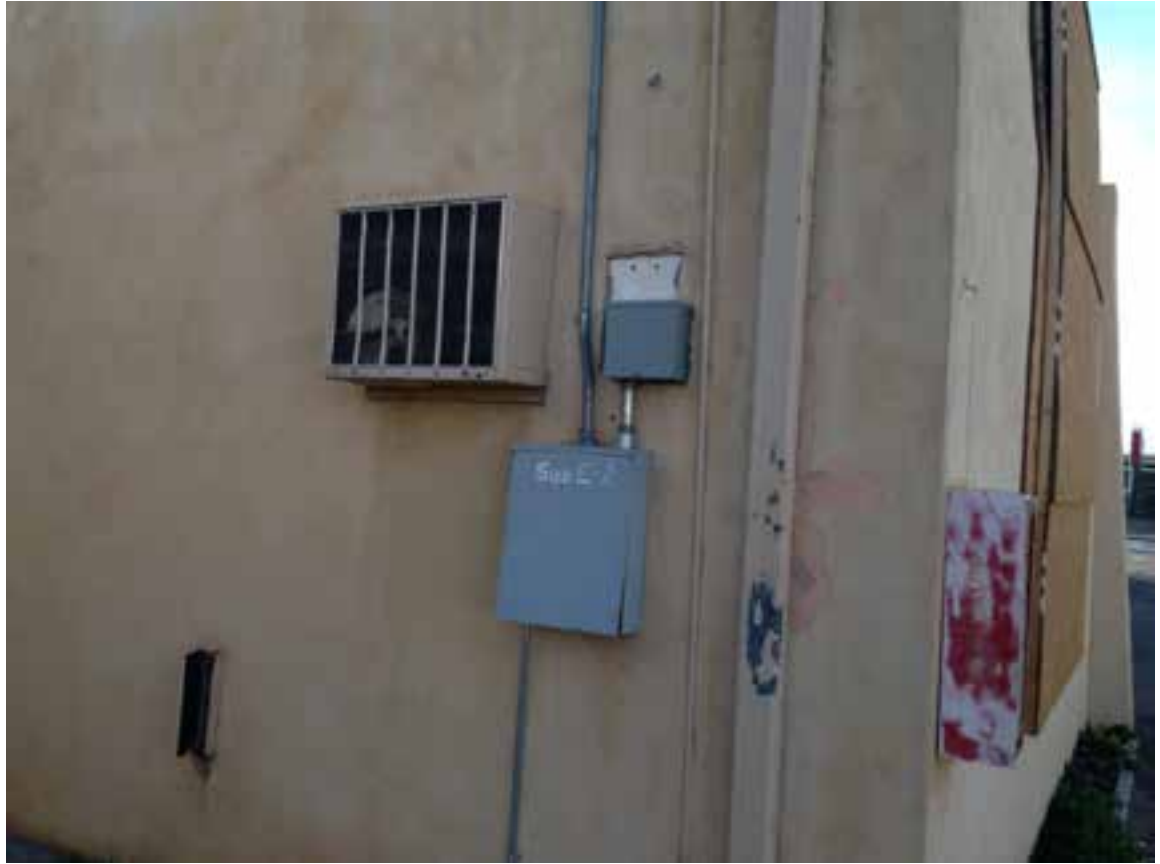
Building “B”– Sub Panel “E1” Mounted On The South Exterior Wall Of Bldg. “B”
