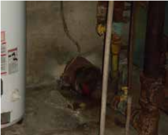
System Distribution Pump
