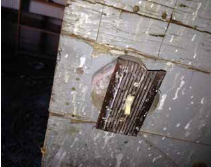
All Hotel Guest Rooms Lighting Controlled With Toggle Switch located at door entrance
