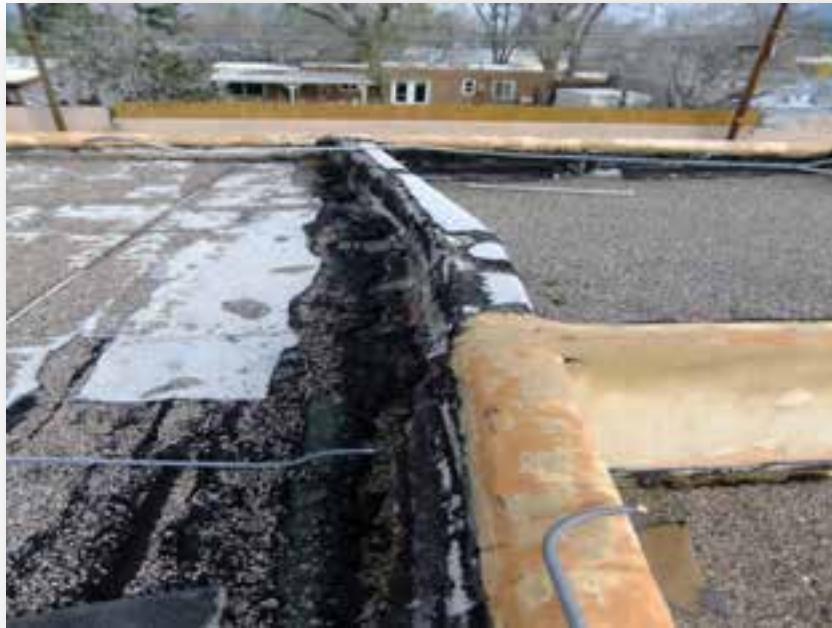
Figure 40 – Building F Distortion at Unit 159
