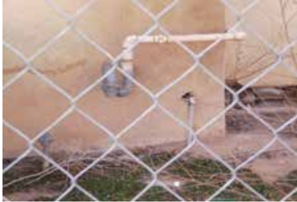
Missing Kitchen Natural Gas Assembly
