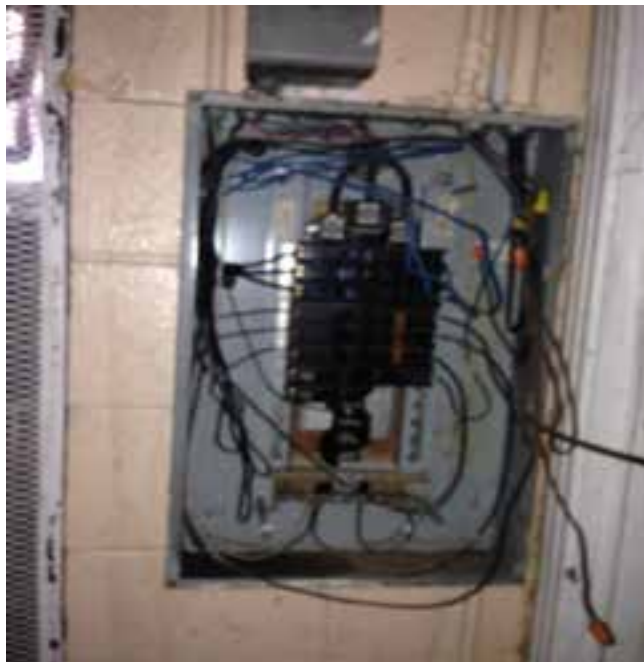
Sub-Panel Located In Hall Of Office Building "E"
