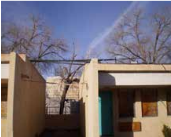
Poorly Supported Natural Gas Piping Between Bldgs F & G
