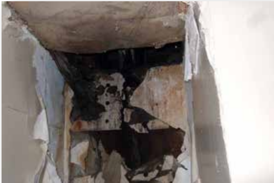
Figure 24- Building D Room 145 Water Damage
