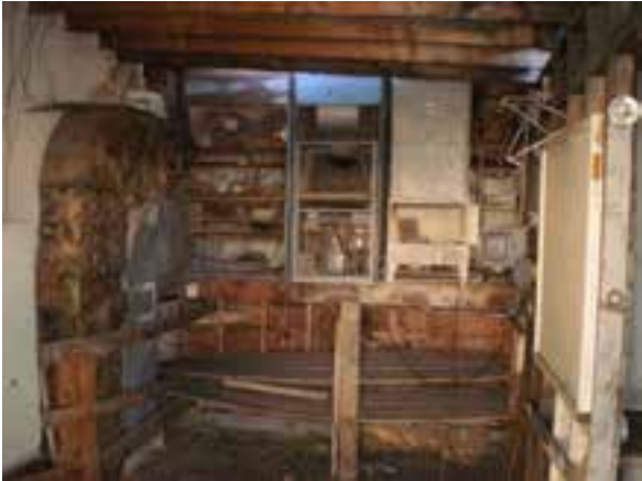
Building 'A' Heating/Cooling System
