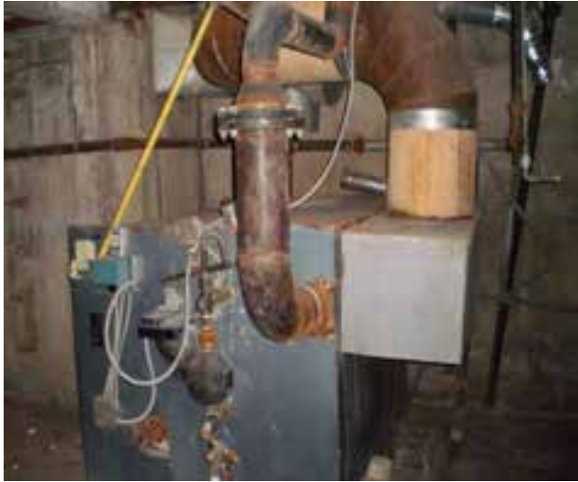
Existing Steam Boiler
