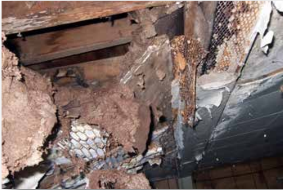
Figure 44- Building G Room 177 Ceiling Collapse
