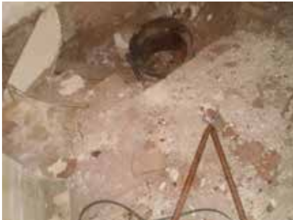
Laundry Room Open Trench Drain
