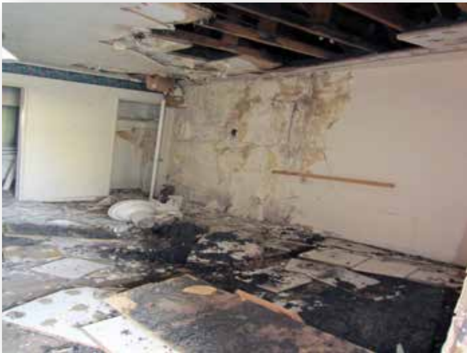
Figure 2- Building A Room 102 Ceiling Collapse
