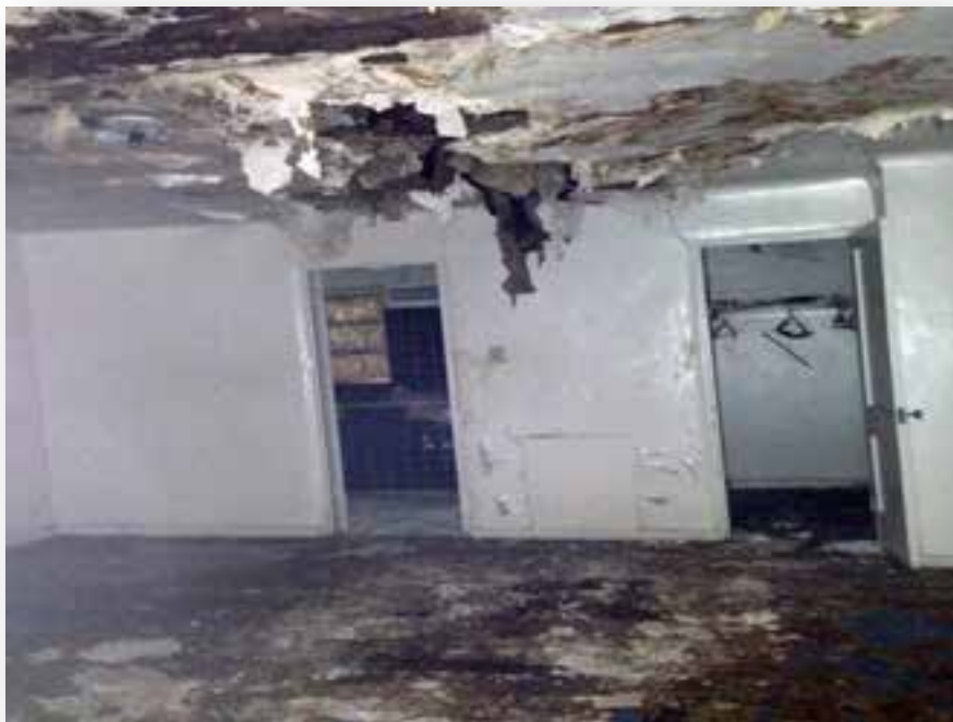
Figure 41- Building F Room 159 Water Damage
