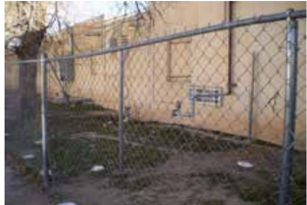
Missing Building Natural Gas Assembly
