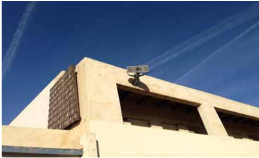
Exterior HID Wall Surface At Various Places On Site
