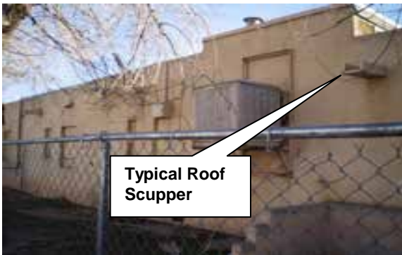
Roof Drainage
