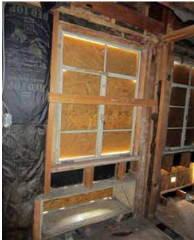
Figure 15- Building B Room 110 - Cut Exterior Studs
