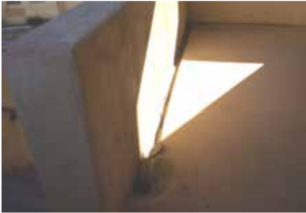
Eastside Landing Drainage
