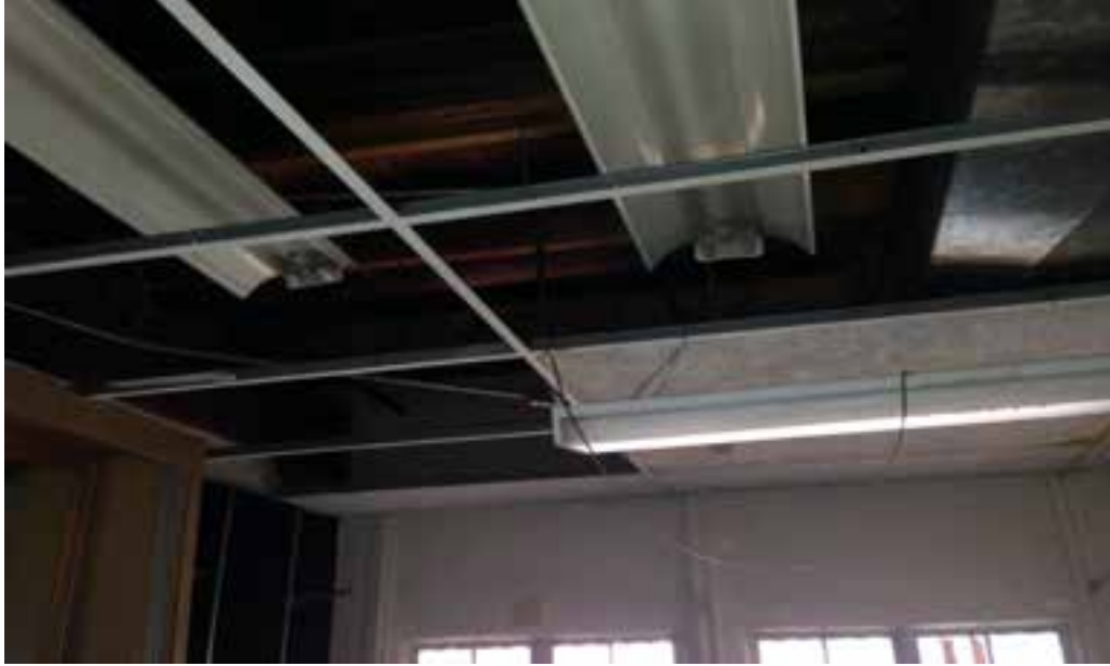
Office light fixtures at Building "E"
