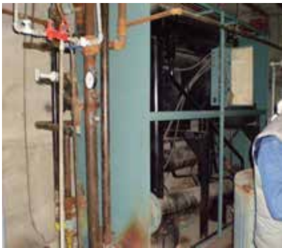
System Water Chiller
