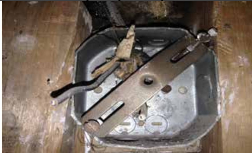
Guest Room Exposed Octagon Junction Box For Lighting At Majority Of Guest Rooms
