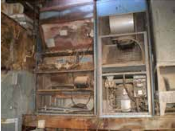
Building 'A' Heating/Cooling System
