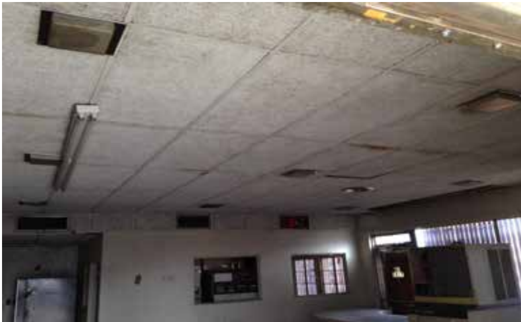
Office Entrance Lobby Area
