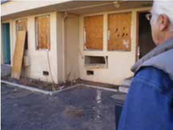
Removed PTAC units without Plywood Cover
