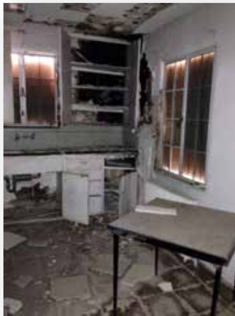
Figure 34-Building E Kitchen Water Infiltration
