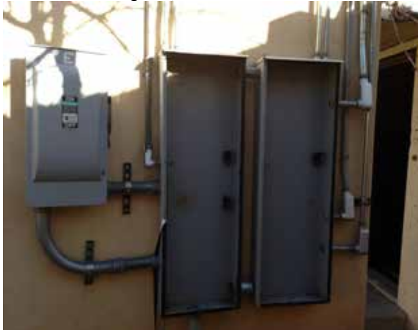
Two Sub-Panels Located At South Exterior Wall Building "B"
