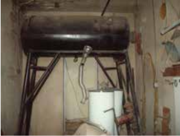
Central Domestic Water Storage Tank
