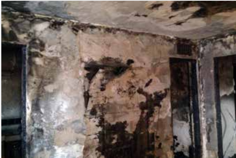
Figure 29- Building D Roof Damage
