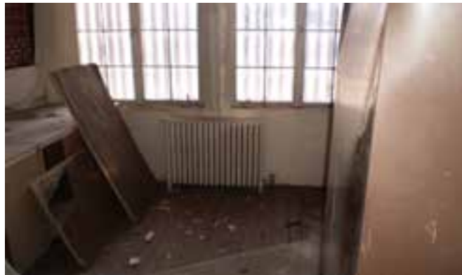
Figure 2 - Typical Steam Radiator with Manual Control
