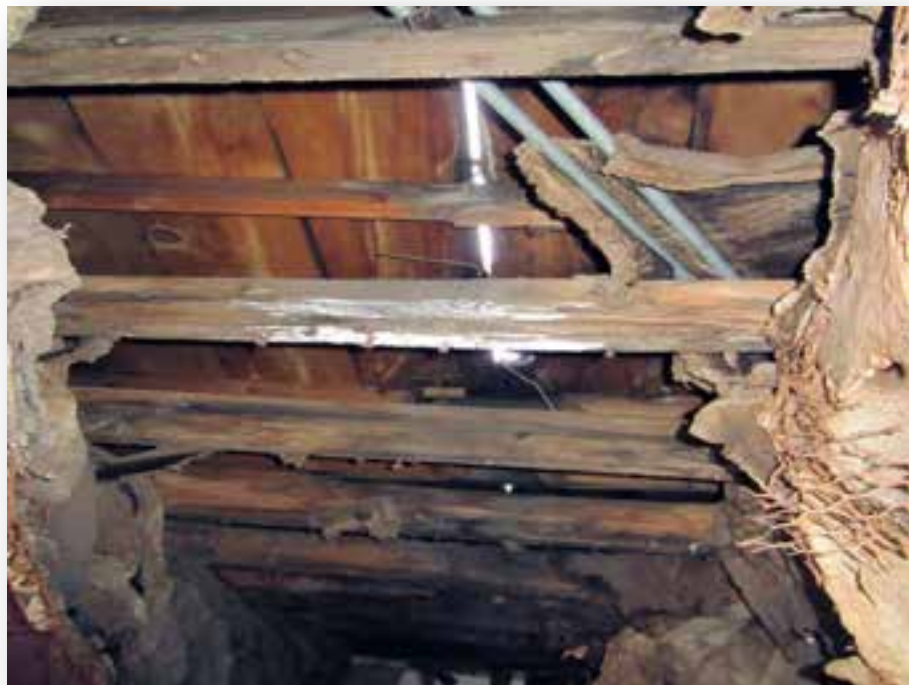
Figure 19- Building C Room 119 Ceiling Collapse at Water Damage
