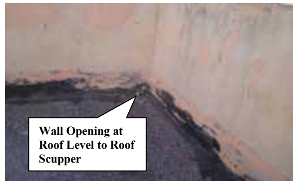
Roof Drainage Lobby East End
