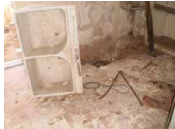
Abandoned Laundry Sink
