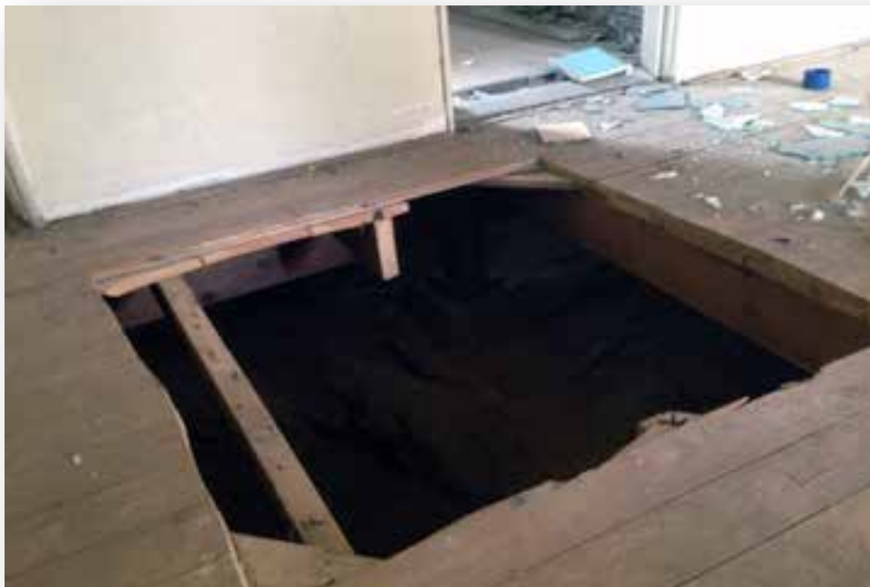
Figure 31- Building D Room 132 Fire Damage
