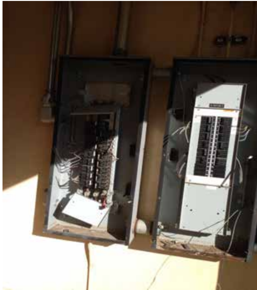
Two Section Sub-Panels Located At South Exterior Wall Building “G”
