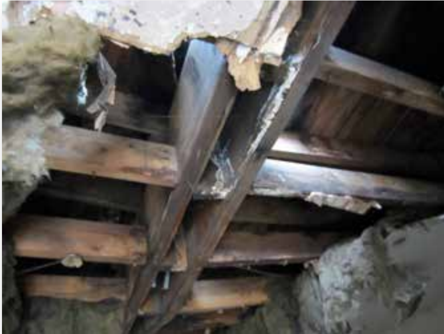
Figure 21- Building C Room 119 Fire Damage – Unsupported Roof Beam
