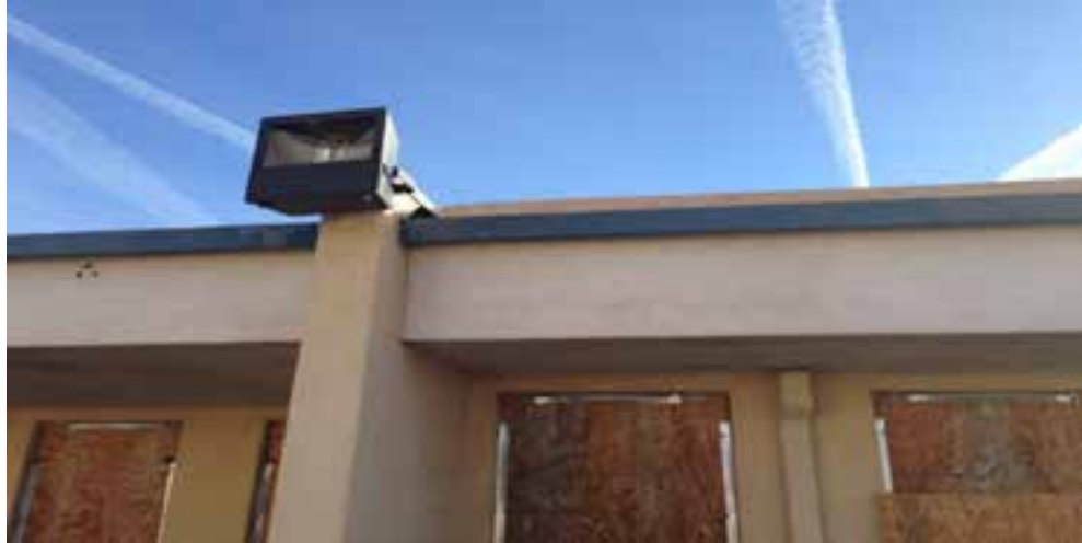
Exterior HID Surface Mount At Various Places On Site
