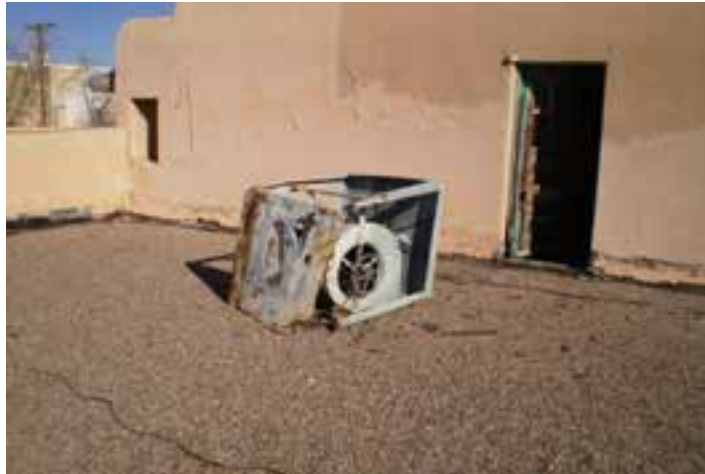
Abandoned Evaporative Cooler for Lobby
