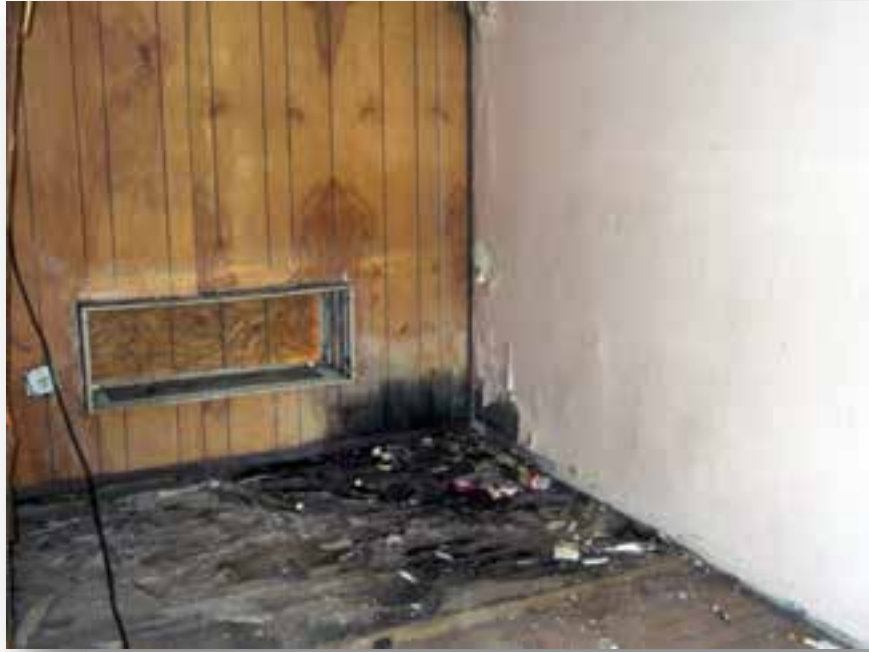
Figure 5- Building A Room 105 – Floor Water Damage
