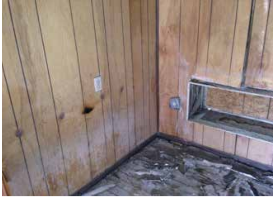
Guest Room Side Wall Heating/Cooling Unit Receptacle With Surface Mount J-Box
