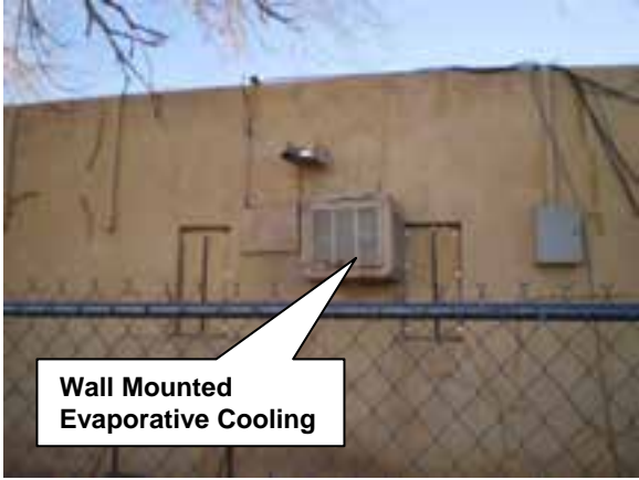
Added Building 'F' Evaporative Cooler
