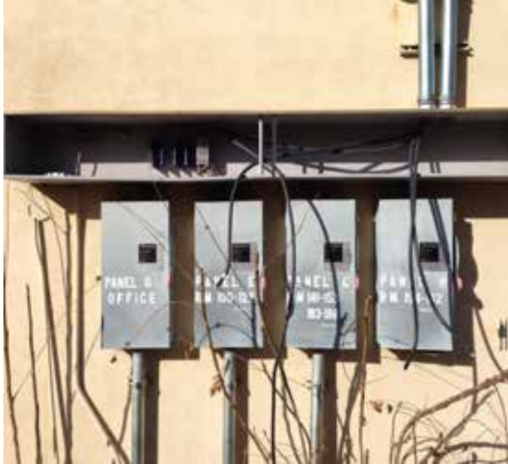
Four Fused Disconnects at East Exterior Wall Of Building "G"
