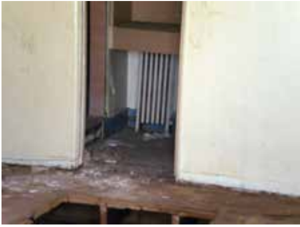
Building D Bath Room Steam Radiator
