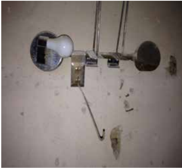
Guest Room Bathroom Incandescent Lighting Fixture and Exposed Conduit
