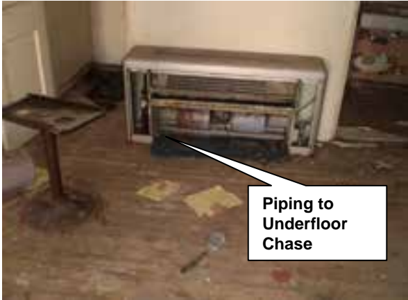
Room Chilled/Hot Water Fan Coil Unit
