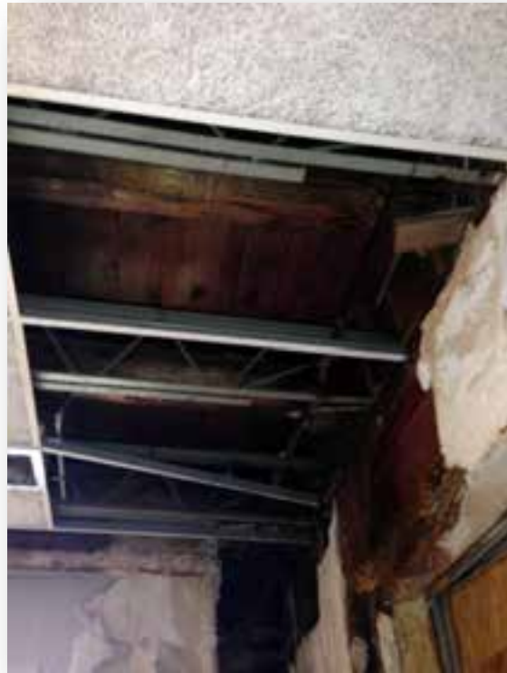
Figure 33- Building E – Lobby - First Floor Ceiling
