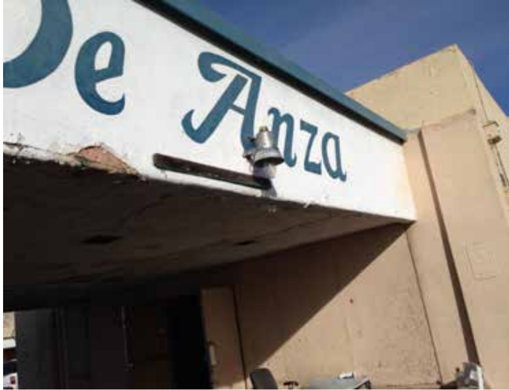
De Anza Entry To Office Lobby with HID Surface Mount Fixtures
