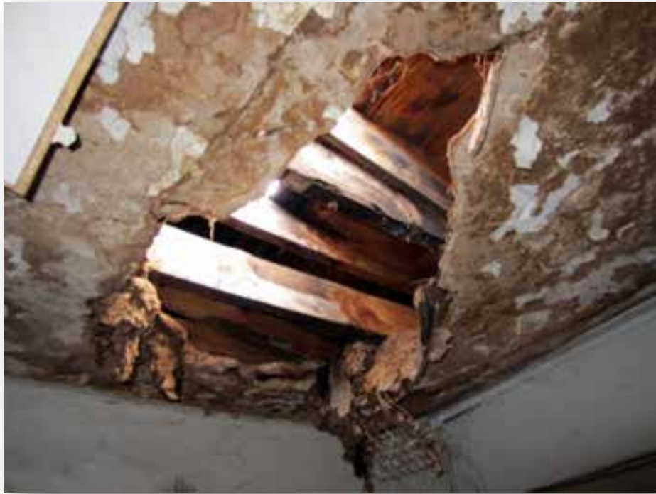
Figure 7- Building A Room 106 – Ceiling Collapse – Exposed Structure
