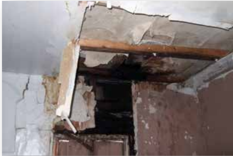
Figure 42- Building G Room 171 Water Damage
