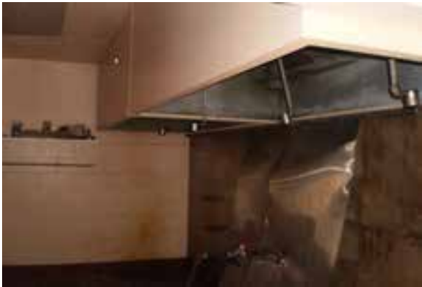
Kitchen Range Hood
