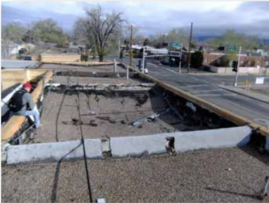
Figure 17- Building C Partially Collapsed Roof Structure
