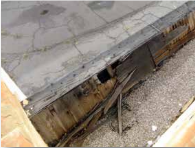
Figure 38- Building F Roof – Missing Flashing
