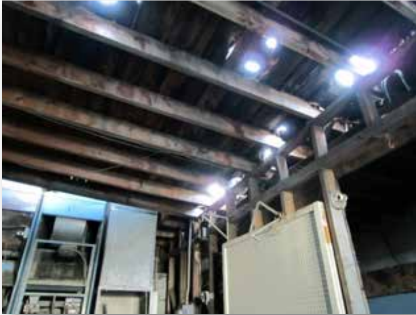
Figure 3- Building A Room 103 – Fire Damaged Room
