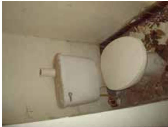
Typical Tank Type Water Closet
