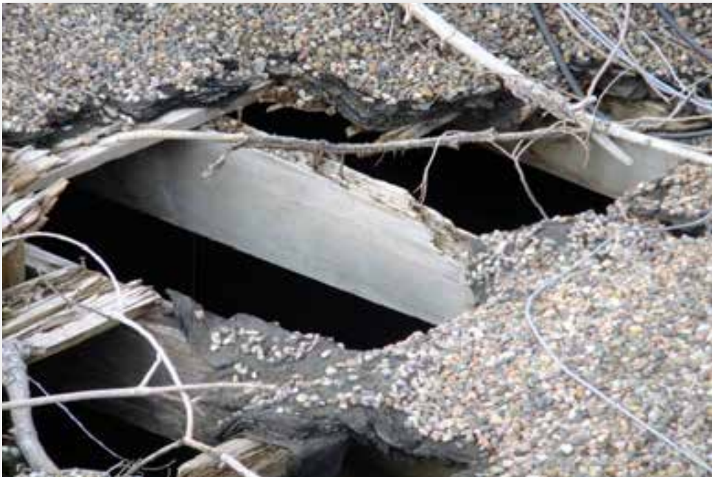
Figure 47-Building G Roof Structure Deterioration
