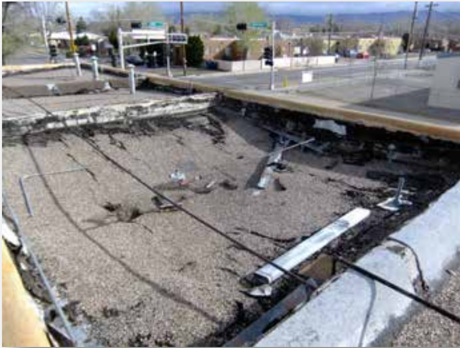
Figure 17- Building C Partially Collapsed Roof Structure
