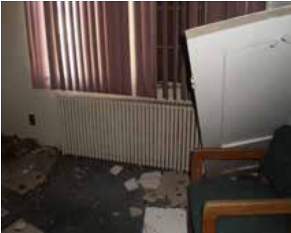
Room Steam Radiator – Manual Control
