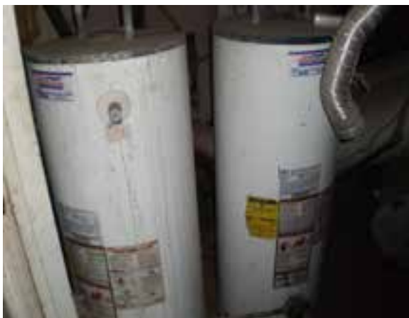
Natural Gas Central Domestic Water Heaters
