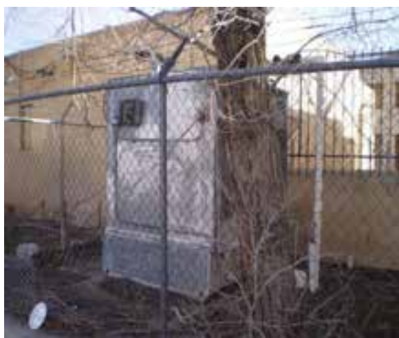
Water Chiller Cooling Tower
