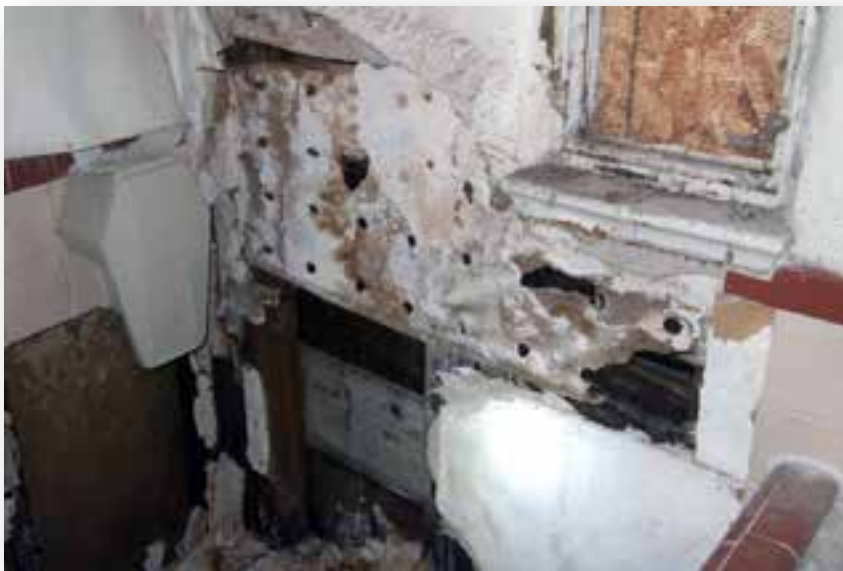
Figure 43- Building G Room 174 Water Damage
