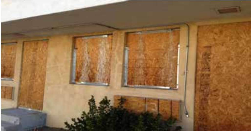
Building “B”– West Exterior Wall Of Bldg. “B”
