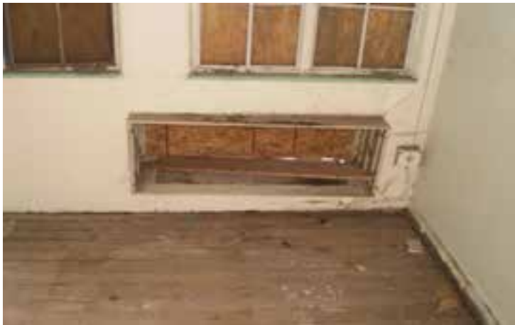
Typical Location of Removed PTAC
