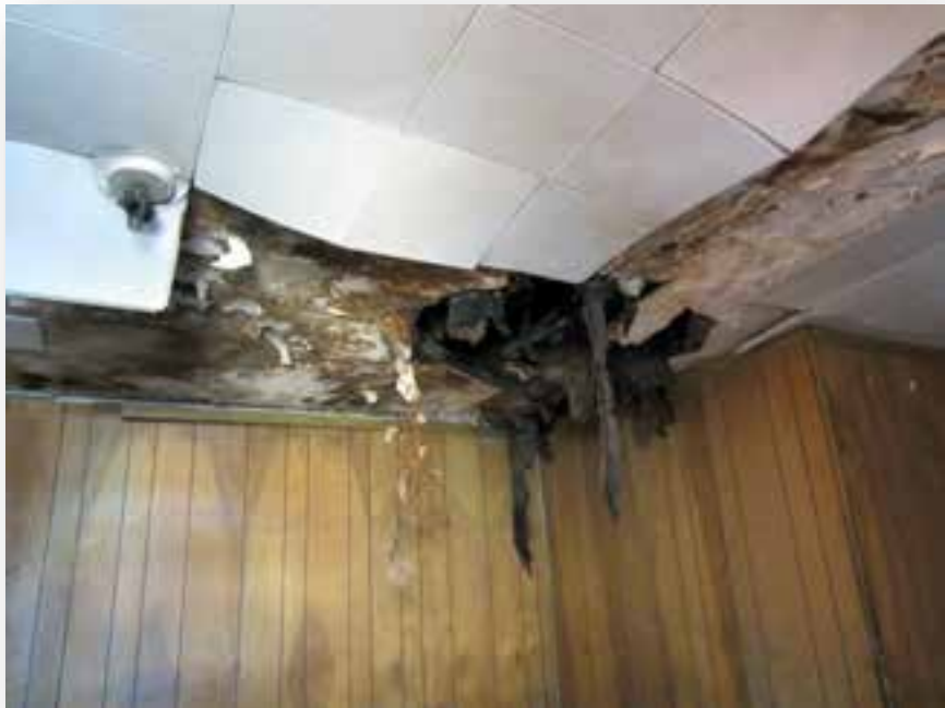
Figure 6- Building A Room 106 – Ceiling Collapse
