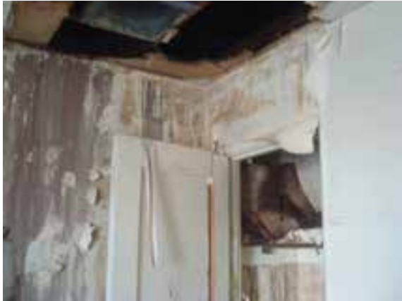
Building 'A' Ceiling Diffuser
