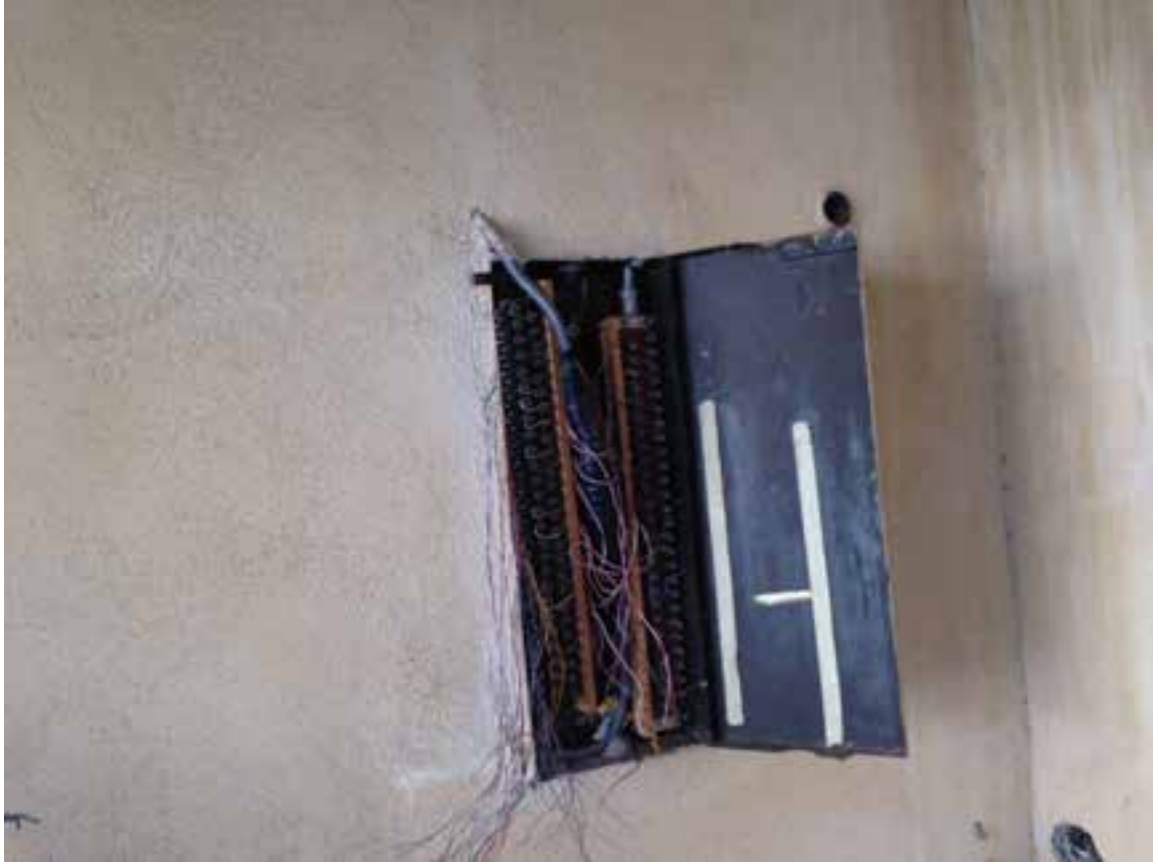
Telephone Terminal Cabinet At South Exterior Wall Of Bldg “B”
