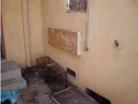
Removed PTAC units with Plywood Cover
