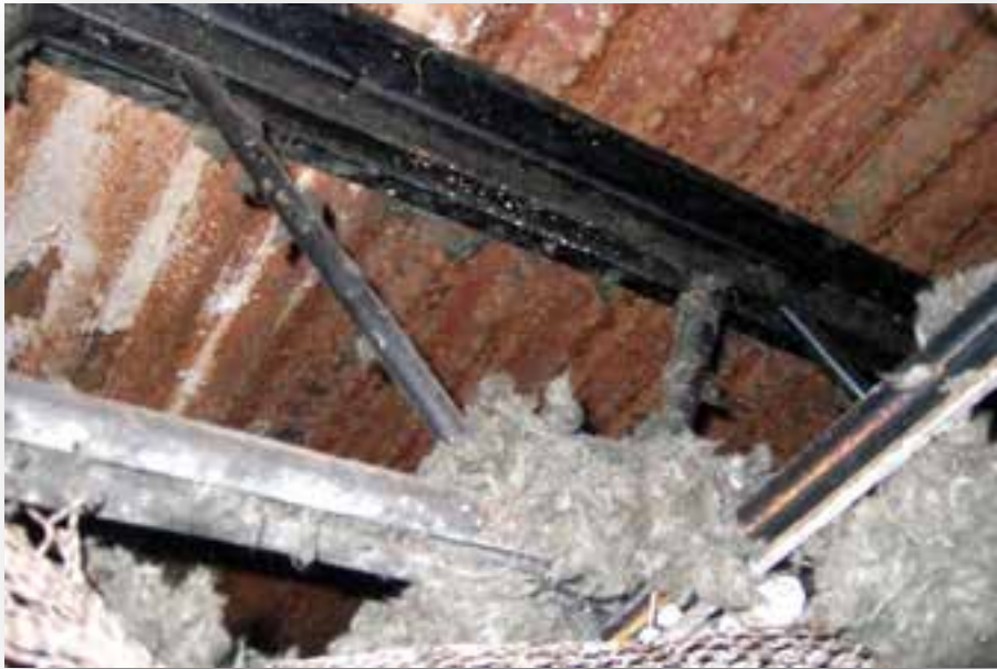
Figure 25- Building D Basement
