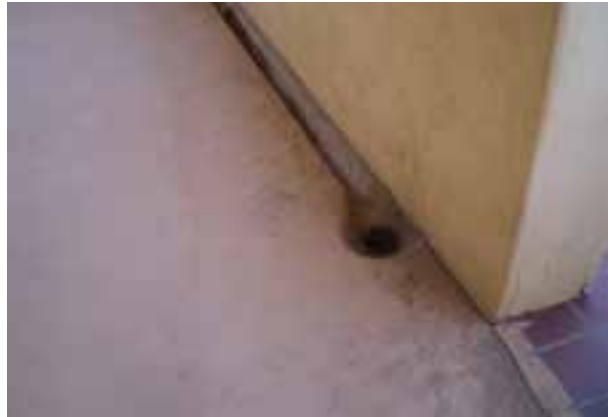
Westside Landing Drainage
