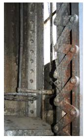
Crank mechanism for skylight operation.
