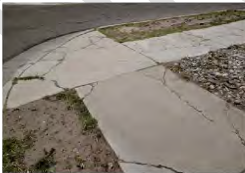
Crumbling sidewalk from shifting land underneath
