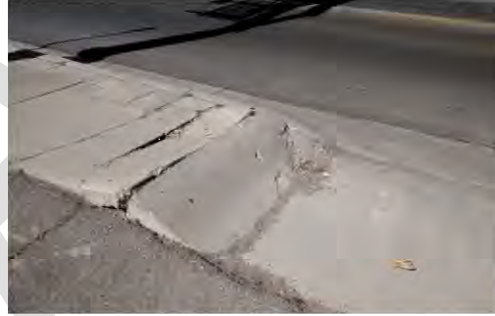
Buckling sidewalk and pavement
