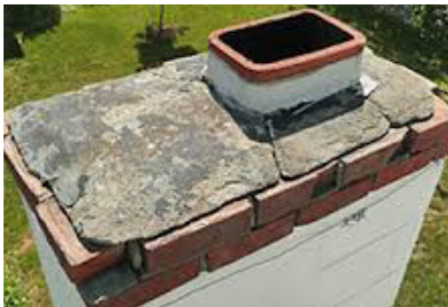
Cracks in chimney
