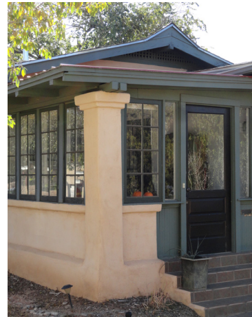
Stucco covered foundation wall
