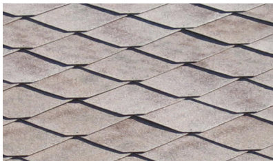
Asphalt shingles - diagonal or "French Method"
