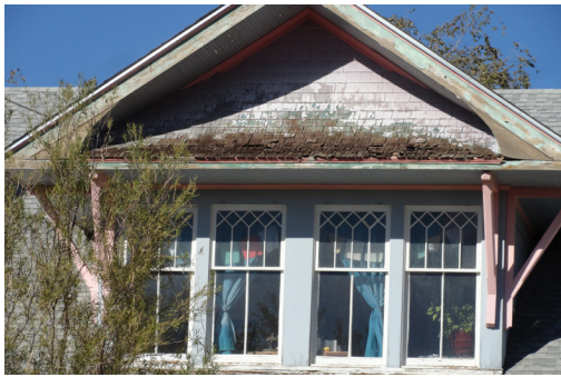
Loose and damaged shingles
