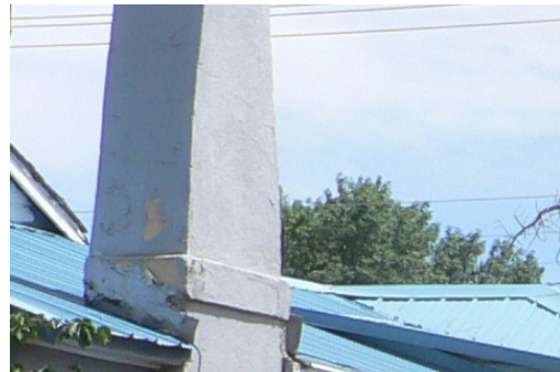
Loose flashing at chimney
