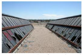
Built-up roofing, positive slope to South.
