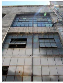
West elevation, Glazing inset to concrete frame.
