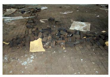
Damaged flooring, 3" thick creosoted end-grain wood blocks
