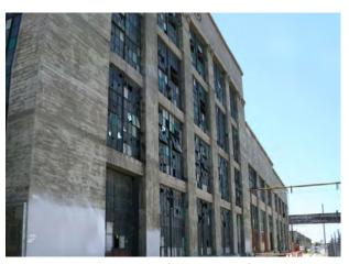
West Elevation, Cast in Place Concrete Frame.
