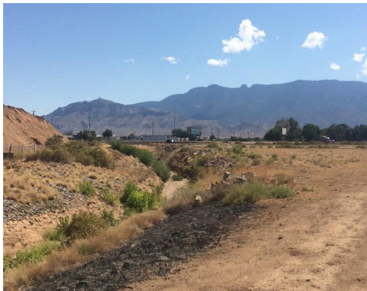
Figure 6 –Deteriorating drainage channel
