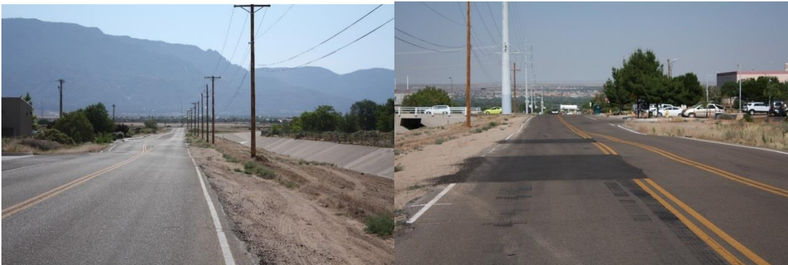
Figure 10 – Existing Conditions along San Diego Avenue
