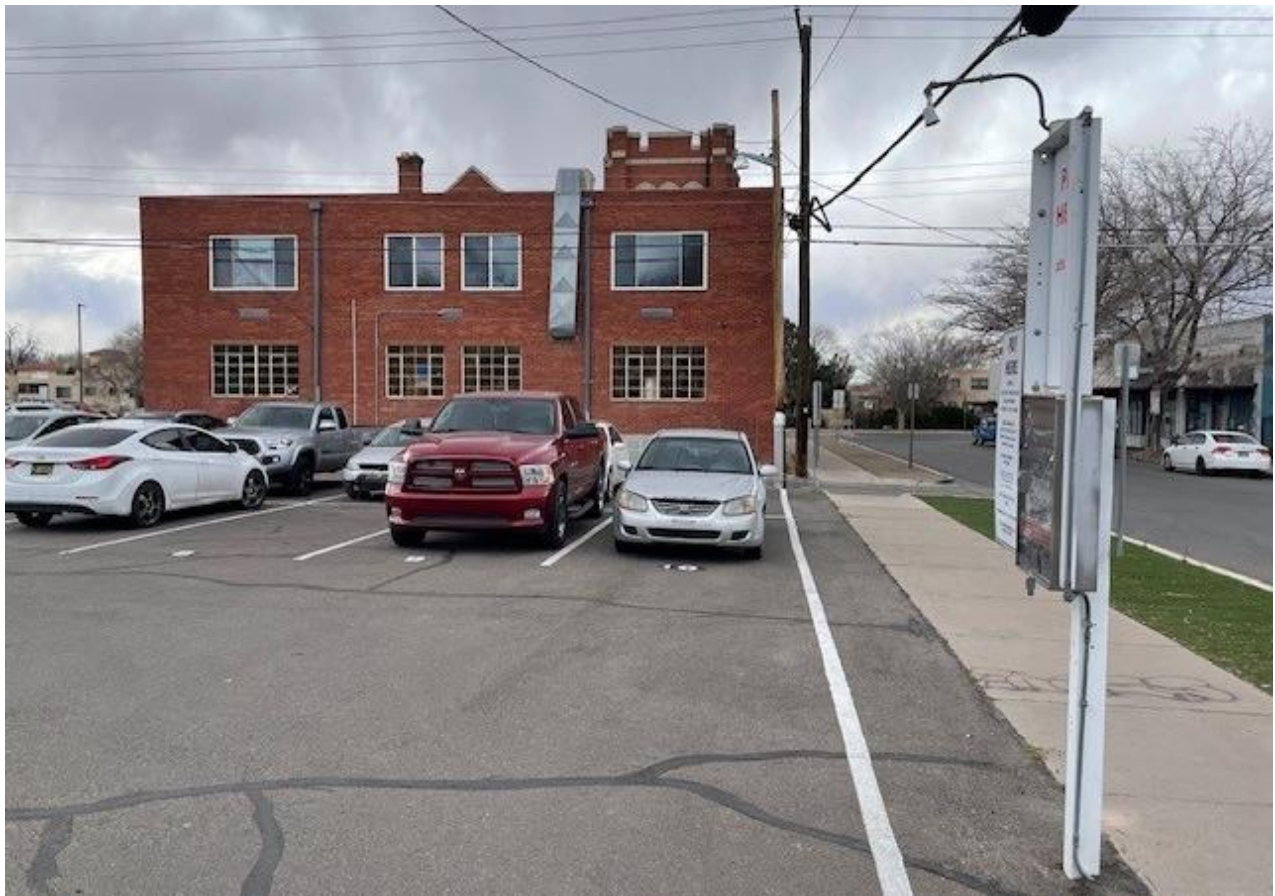
Figure 6: Looking west to rear parking lot of 201 & 203 Harvard Dr. SE and church on Yale SE.
