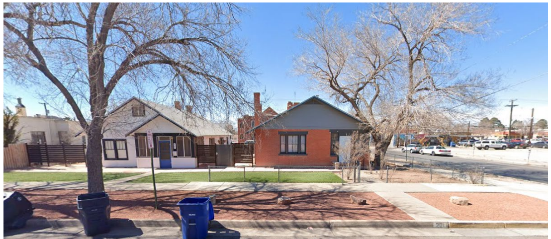
View looking west to the subject property
