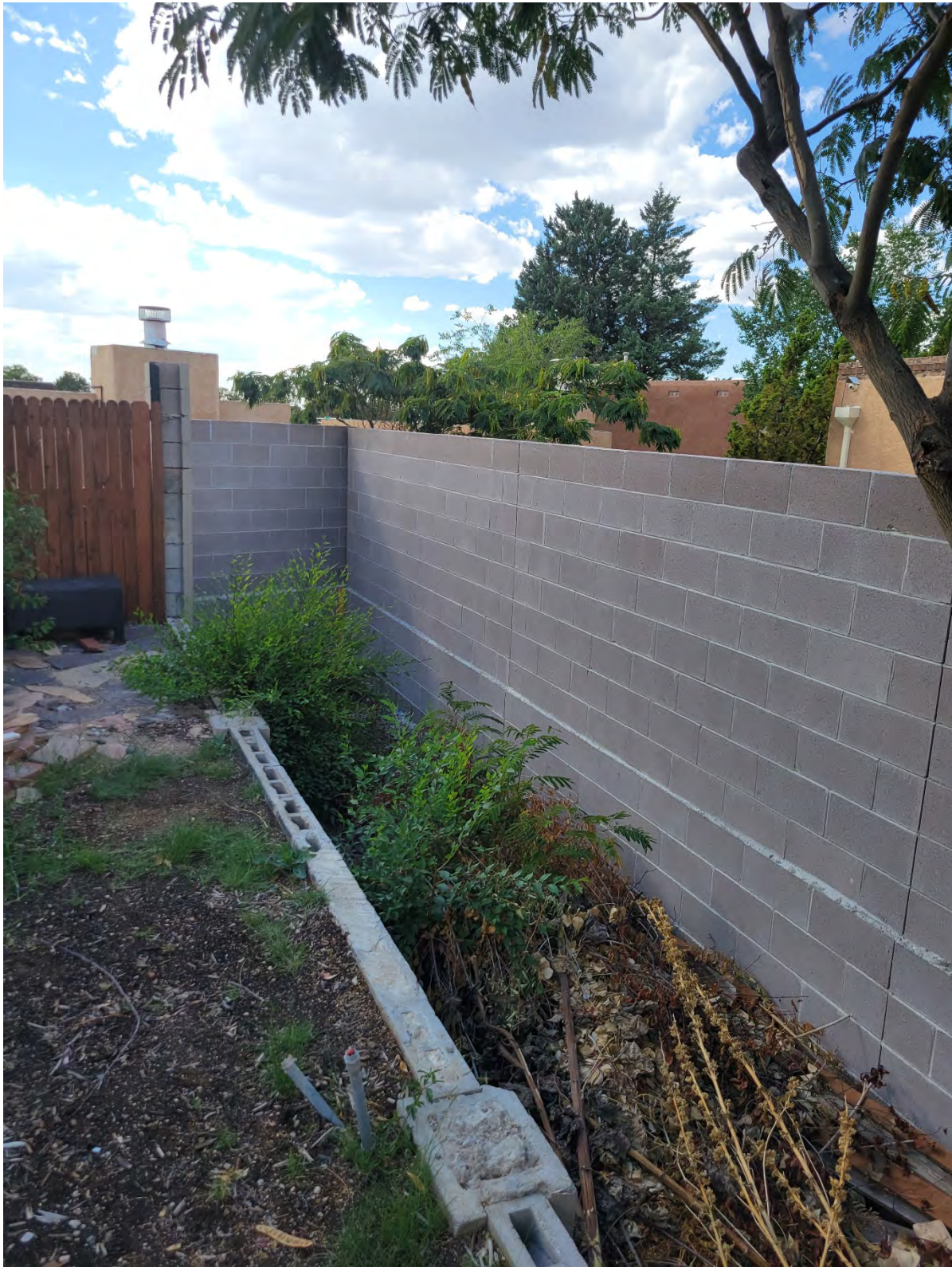
Figure 1 - Extended CMU Block Retaining Wall with Existing Secondary Wall
