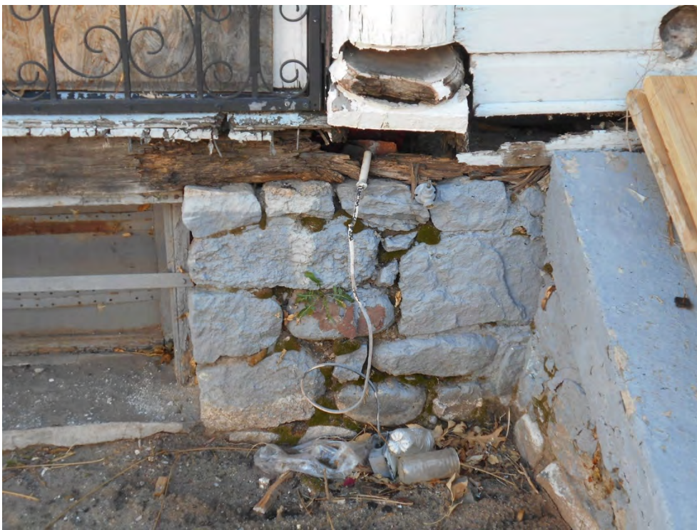
Rear floor structure and column damage.
