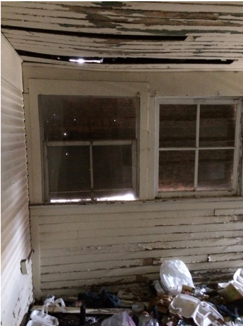
Second level porch and roof damage.
