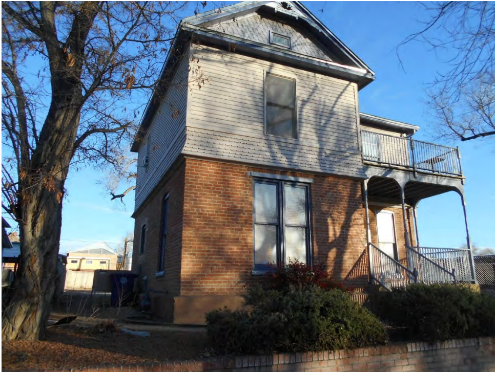
Typical frame over brick construction and flair between stories at 112 Edith NE
