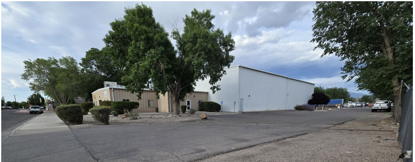
Figure 2: Overview of subject site - looking NE.
