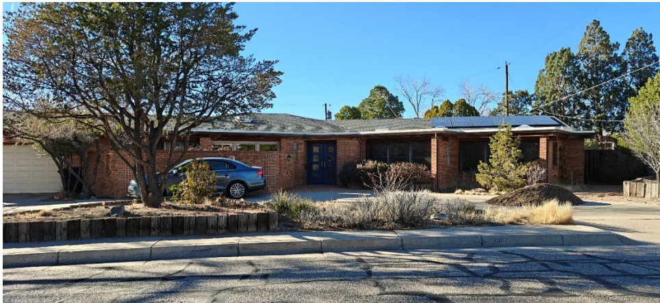
14-16-6-6(H)(3)a: Below photos demonstrate two properties with walls over 3 feet in height in the front yard.
