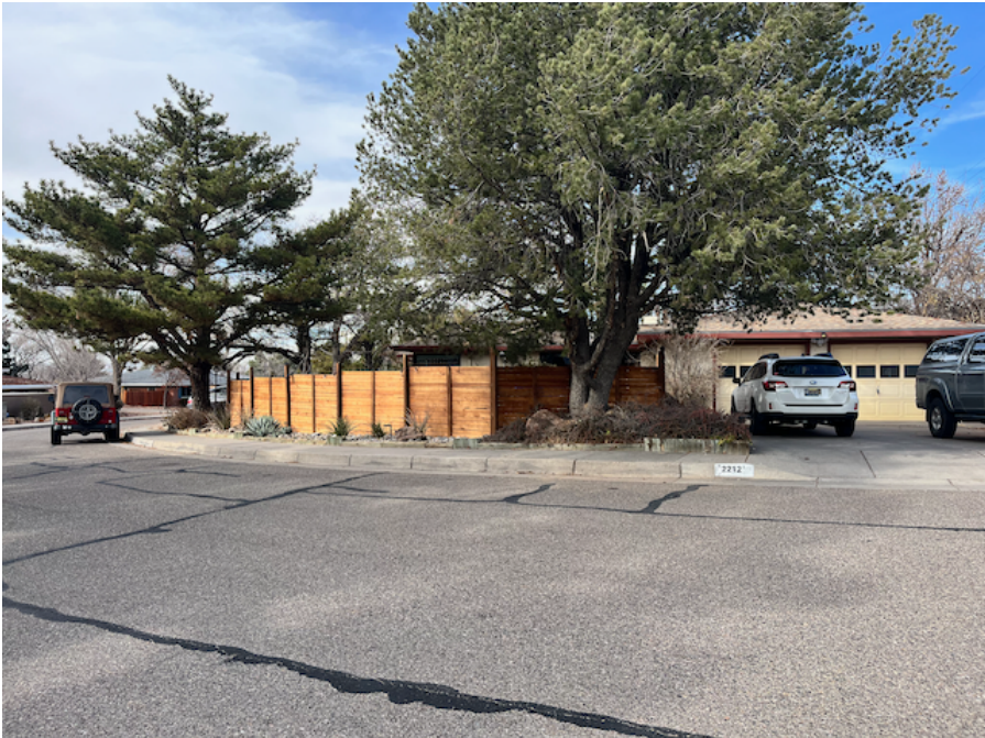
Figure 2: Side of house
