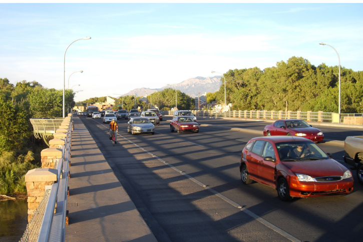
The Central Ave. Bridge crossing the Rio Grande serves all travel modes.
