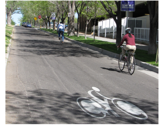
There are many types of bike facilities that are appropriate for different roadways and contexts. Protected bike lanes are important where cyclists are close to traffic, while bike boulevards are more appropriate in low-traffic areas.
