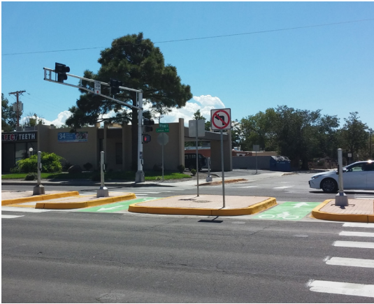
Signalized bike and pedestrian crossings with a median refuge and well-marked bike lanes make it safe and easy to travel the city by bike and cross busy streets.
